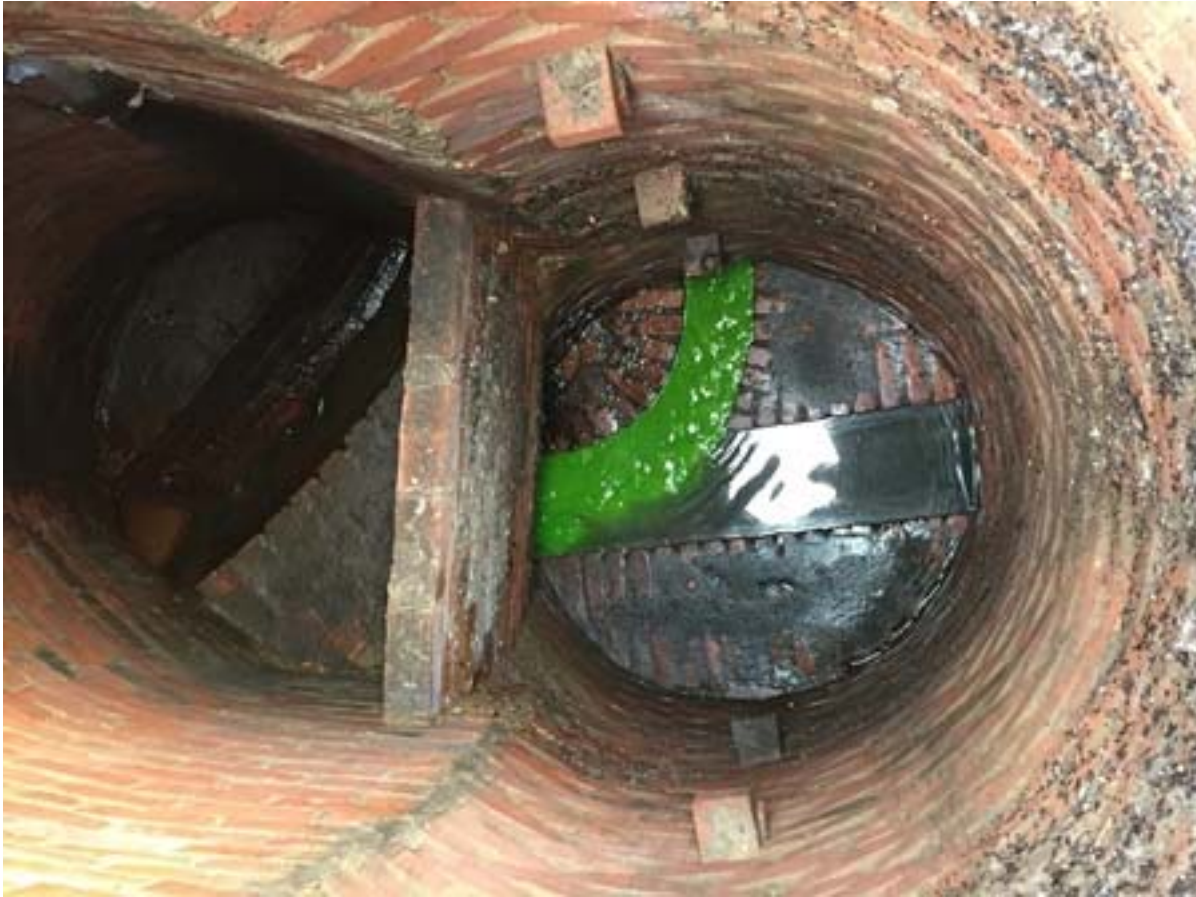
Figure 7 Sanitary Connection to Tannery Brook System
