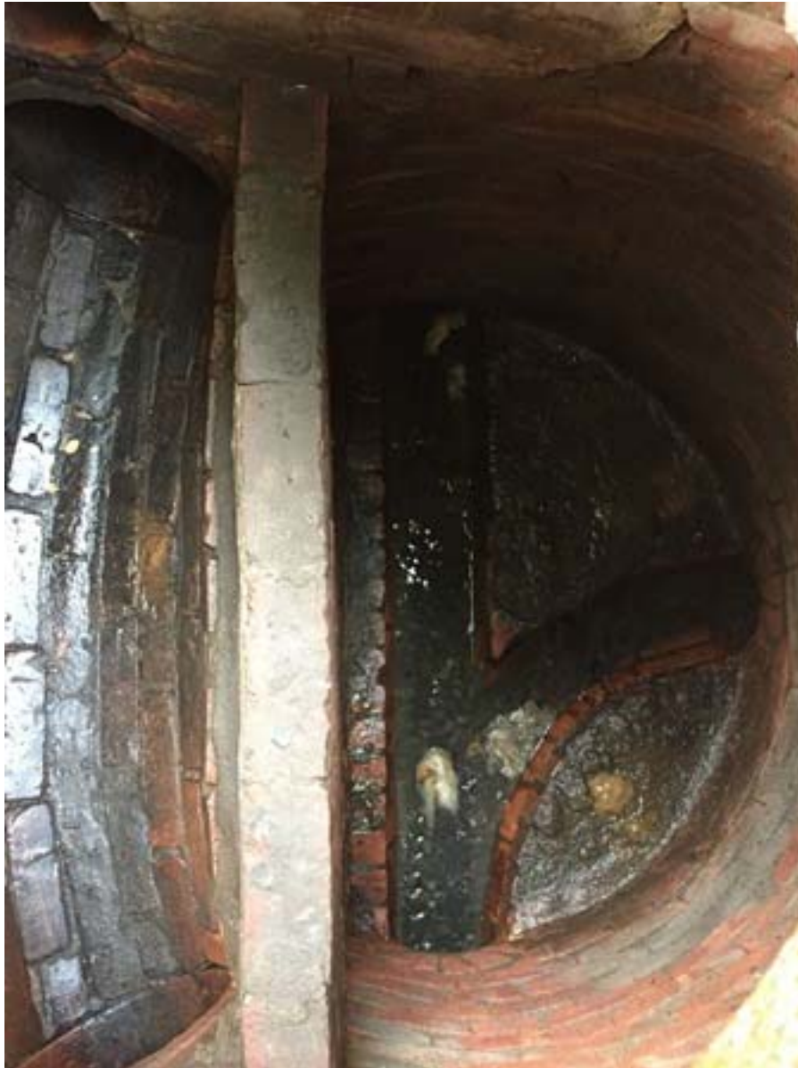
Figure 4 Sanitary in Common Manhole
