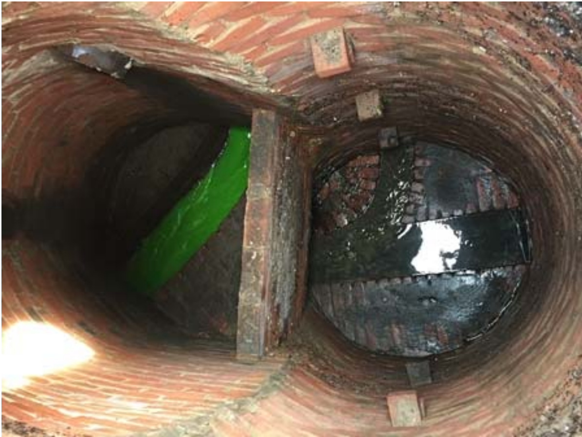
Figure 8 Storm Connection to Tannery Brook System
