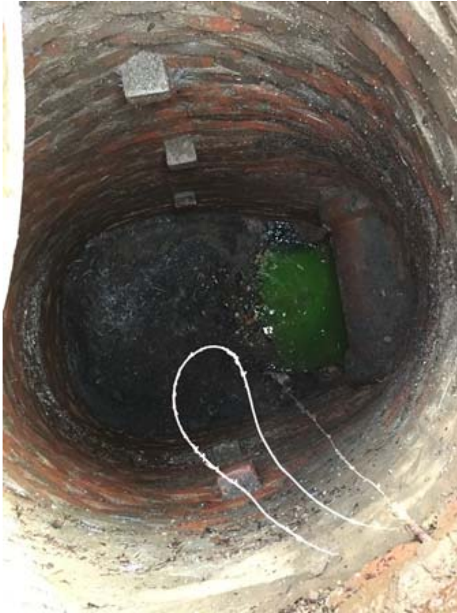
Figure 6 Obstructed Flow near Harrison Road
