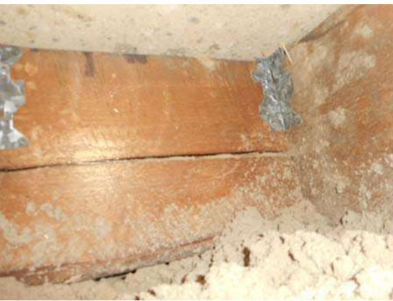
SECOND FLOOR JOIST WITH MODERN LIGHT STEEL ANGLES INDICATING RECENT FLOOR REPAIRS.
