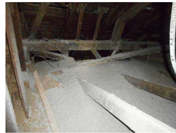
TIMBER PURLIN ALONG ROOF SET BACK FROM EAVE SUGGESTS A FORMER STAIR OPENING WITHIN THE GABLE ROOF.
