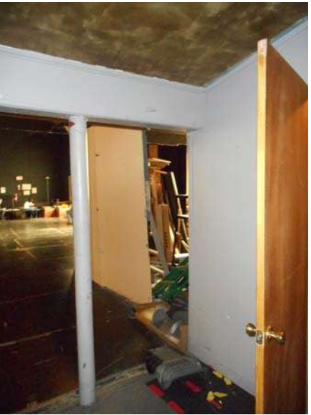
TIMBER BEAM ON PIPE COLUMNS IN BAY NEXT TO ADDITION MAY HAVE BEEN PART OF FORMER STAIRWELL.
