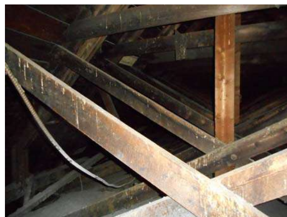
MAIN ROOF IS SUPPORTED WITH STICK FRAMED SCISSOR TRUSSES SPANNING OVER HALL TO EXTERIOR WALLS.
