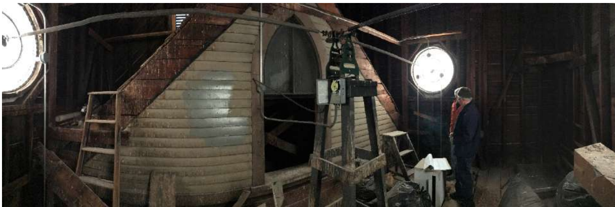
7 Panorama view of the interior of the clock tower showing the end gable of the original church. The geared mechanism to run the clocks is to the right of the ogee window. Note also the crossed-braced framing in the exterior walls.
