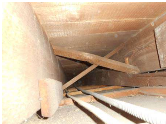
FIRST FLOOR JOISTS SUPPORTED ON TIMBER BEAMS
