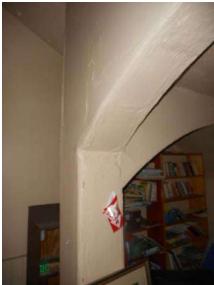
CONCEALED ARCH FRAMING NEXT TO ADDITION SUGGESTS A FORMER STAIRWELL IN ORIGINAL BUILDING.
