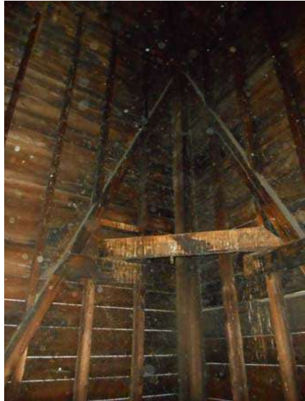
UNBRACED STUD HEIGHT IN TOWER IS EXCESSIVE.
