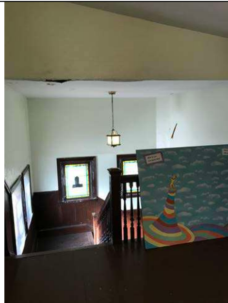
19. Front Hall Stair showing plaster damage from water intrusion.
