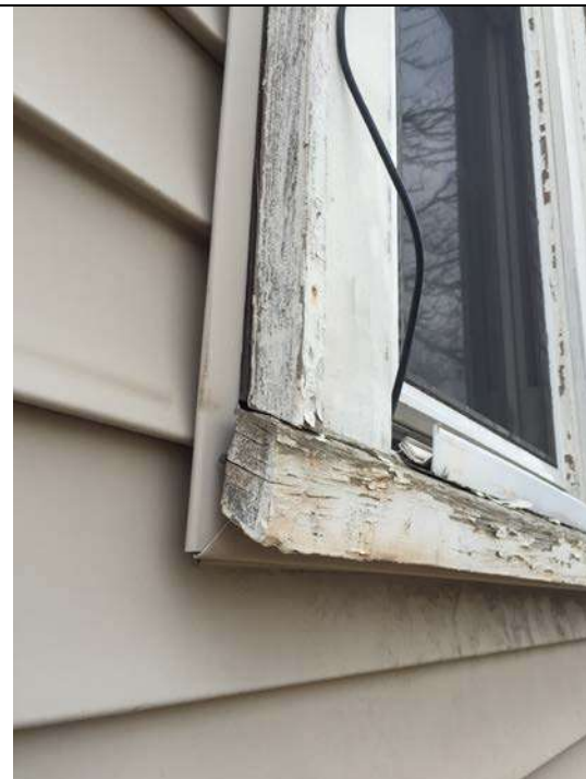
11. Condition of Exterior Window Trim and Sill.
