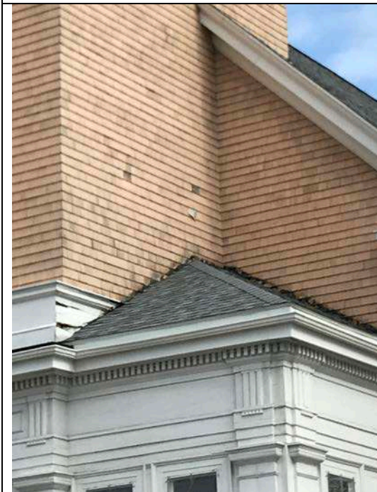
6. Flawed cheek wall flashing
