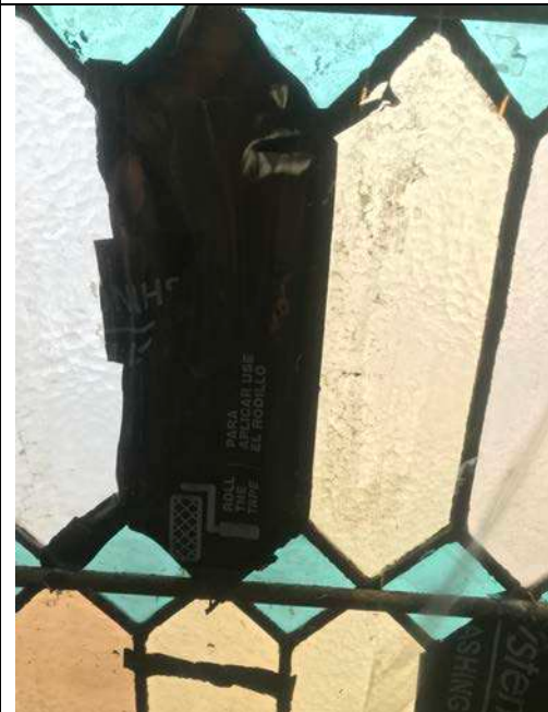
18. Temporary patches on broken Stained Glass Windows
