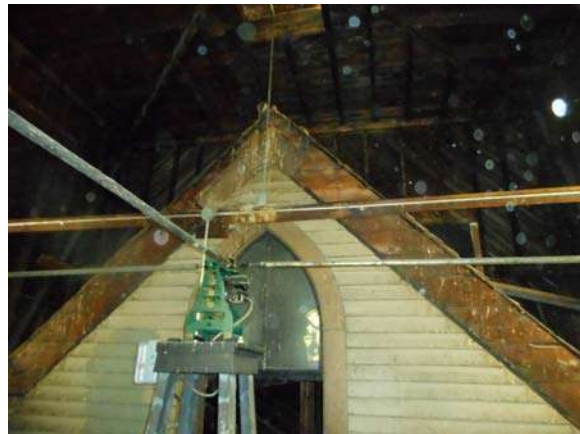
GABLE END OF MAIN ROOF CONCEALED IN TOWER. IT'S EXTERIOR SIDING INDICATES THE TOWER IS AN ADDITION.
