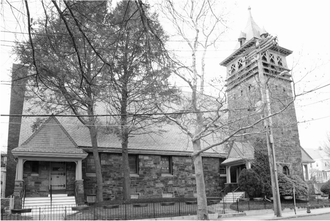
Photo 3. View of left (east) side elevation and corner tower, looking west.
