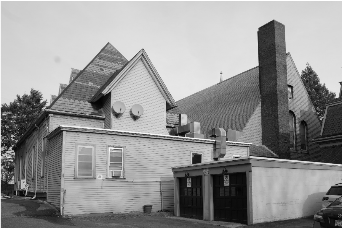
Photo 5. View of rear (south) elevation, looking northeast.
