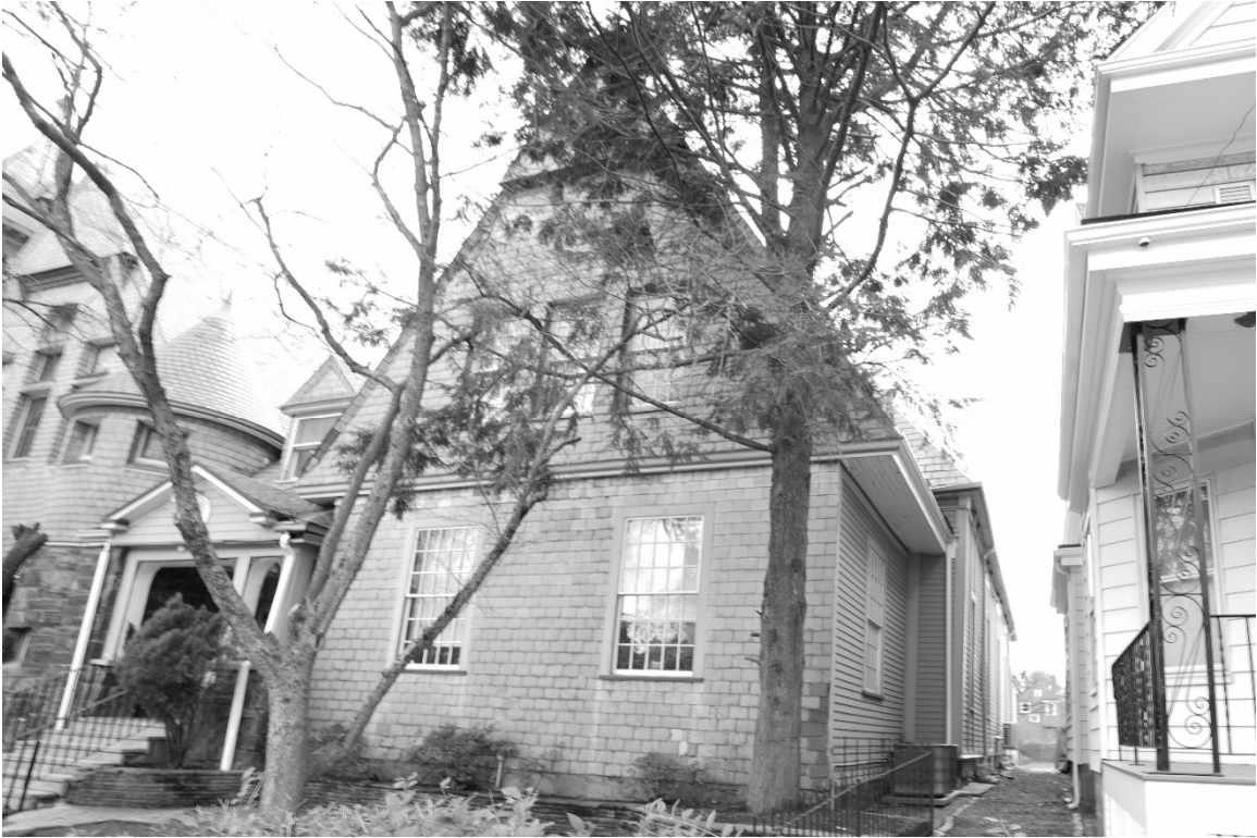
Photo 7. View of front (partial) and right (west) side elevation, looking southeast.
