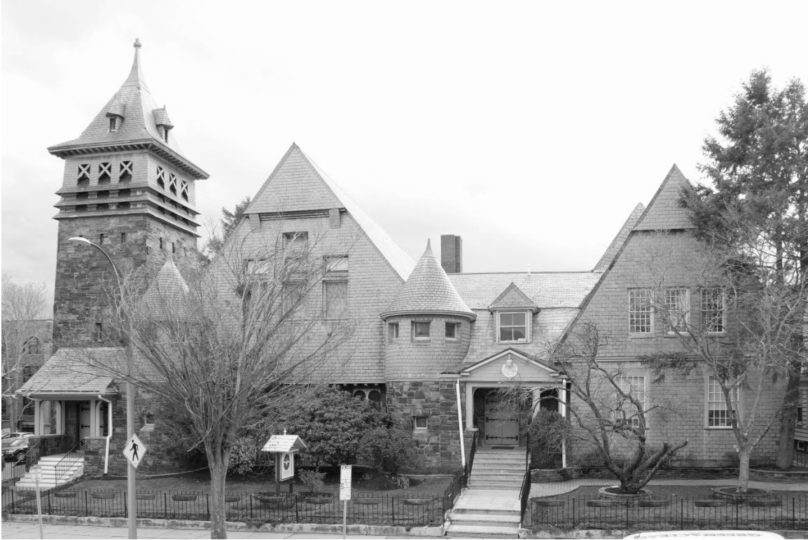
Photo 1. View of front (north) elevation, looking south.
