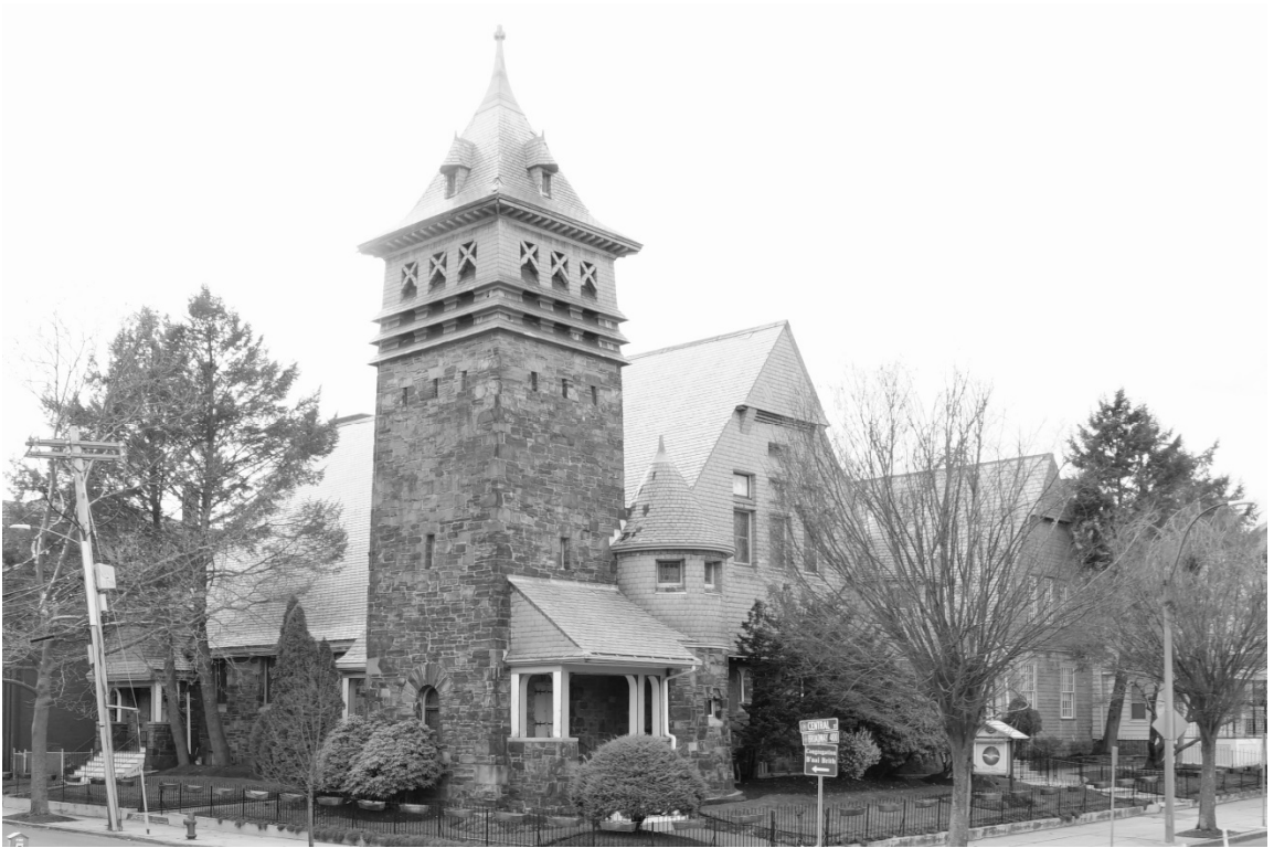
Photo 2. View of front (north) and left (east) side elevations and corner tower, looking southwest.
