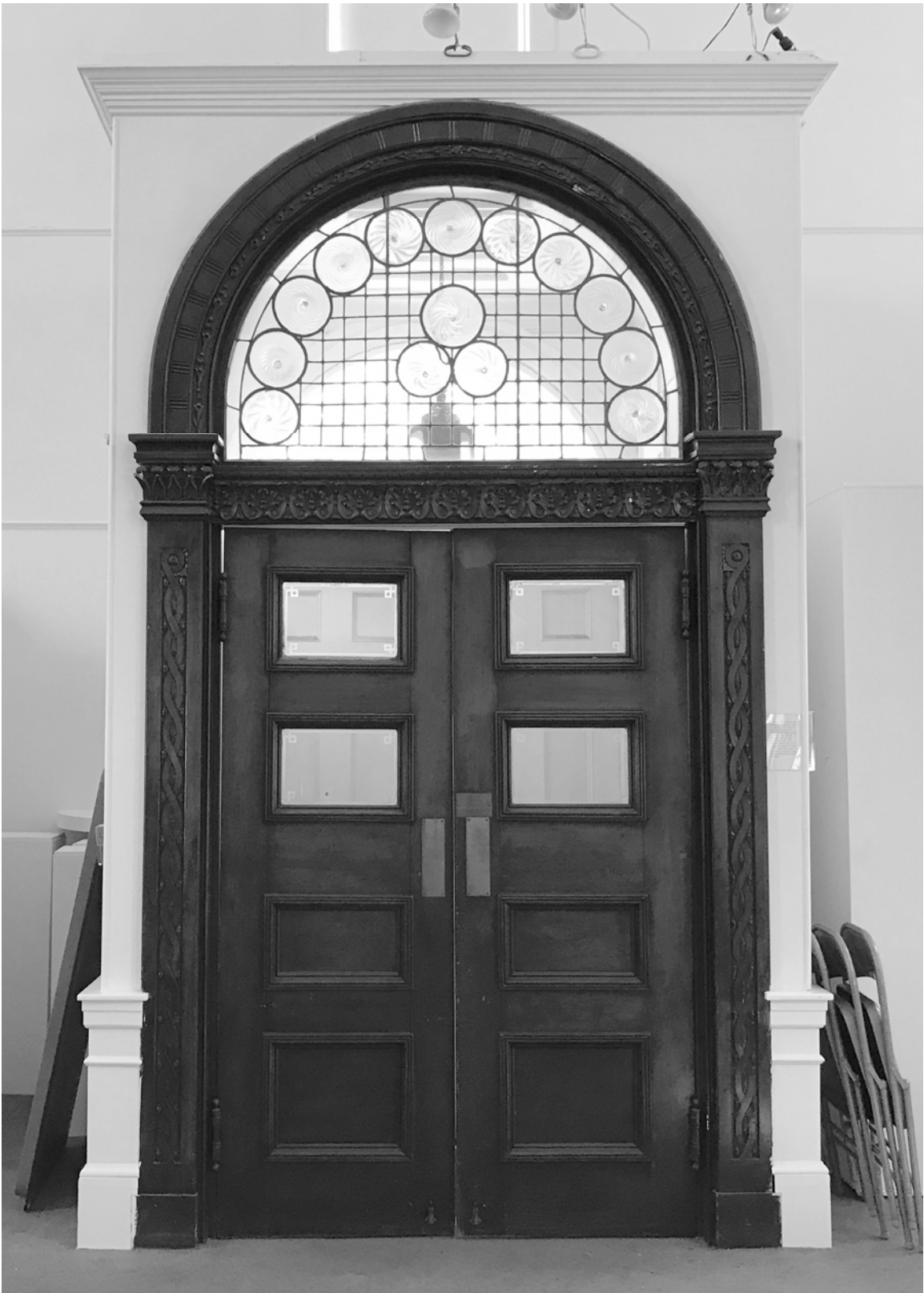
Photo 7. View of interior Loring Library doors, looking southeast.
