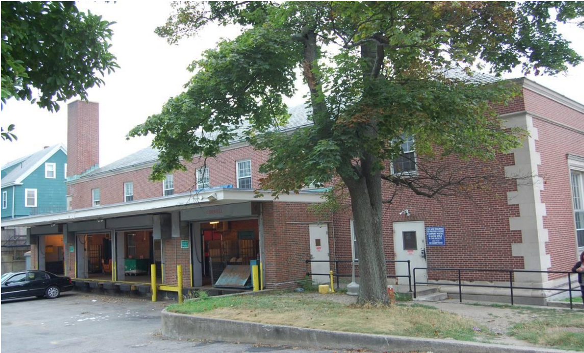
Photograph 3. View of north (rear) elevation looking southeast from Bonner Avenue.
