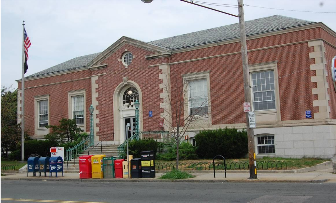
Photograph 1. View of south (facade) elevation looking northwest from Washington Street.
