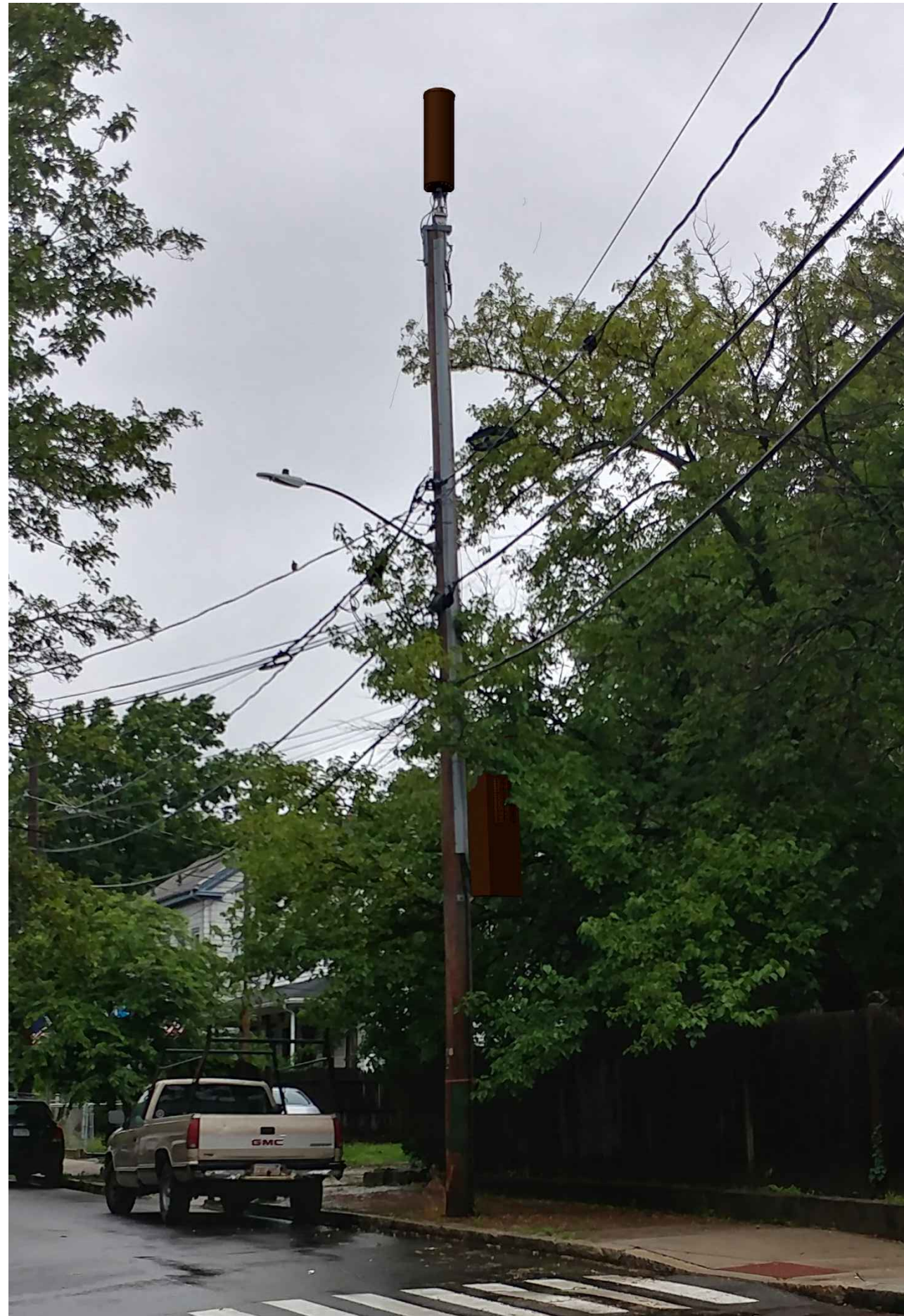
UTILITY POLE – AFTER
