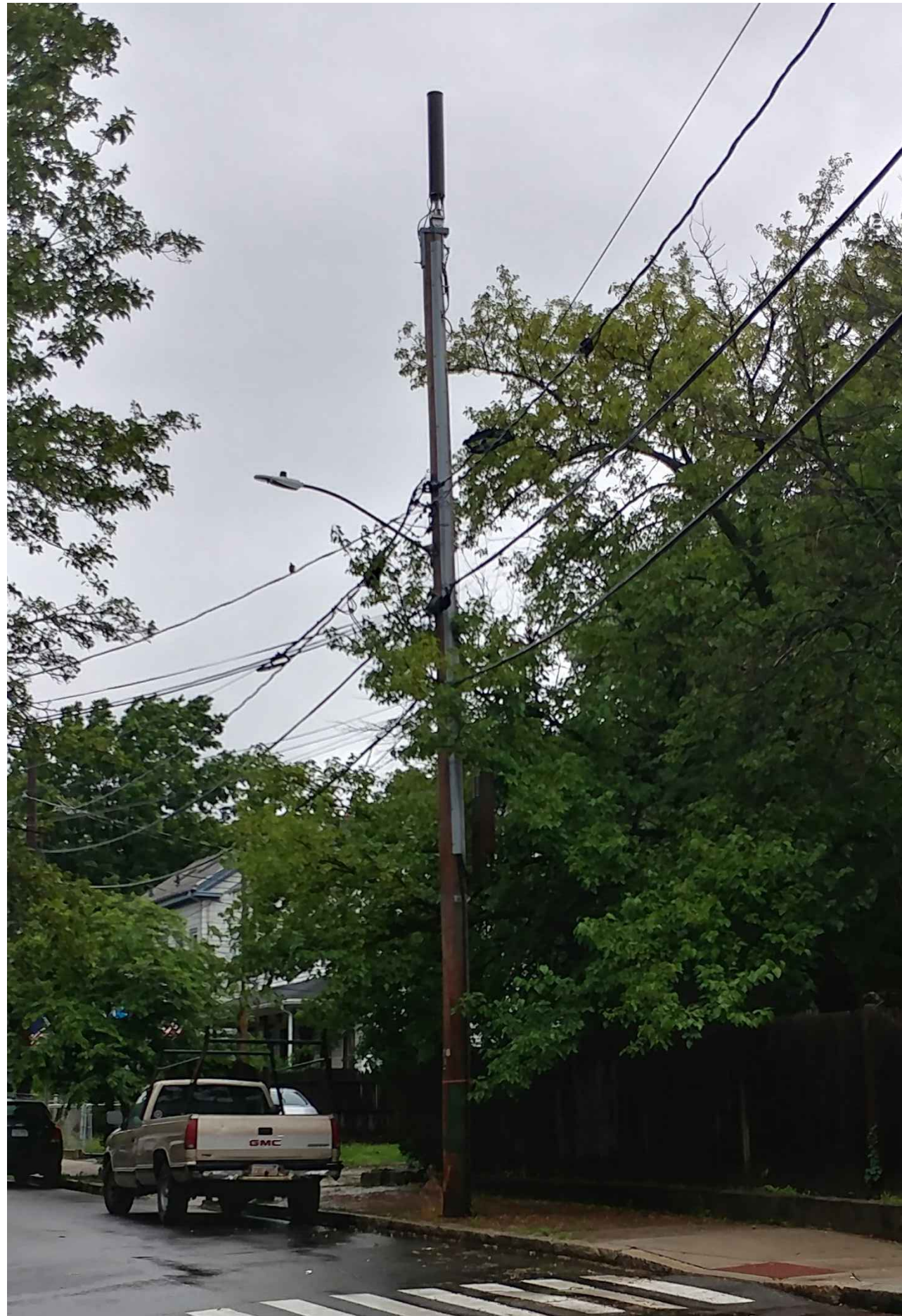
UTILITY POLE – BEFORE
