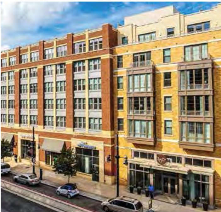
Figure 5.1.11 (a) Appearance of Two Buildings
