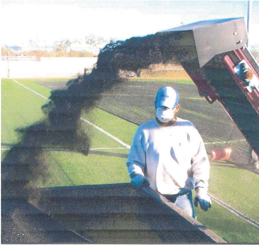
The Turf Industry MSDS warns waste tire installers to wash exposed areas frequently, wear a respirator, wear safety goggles, and remove and wash clothes.
