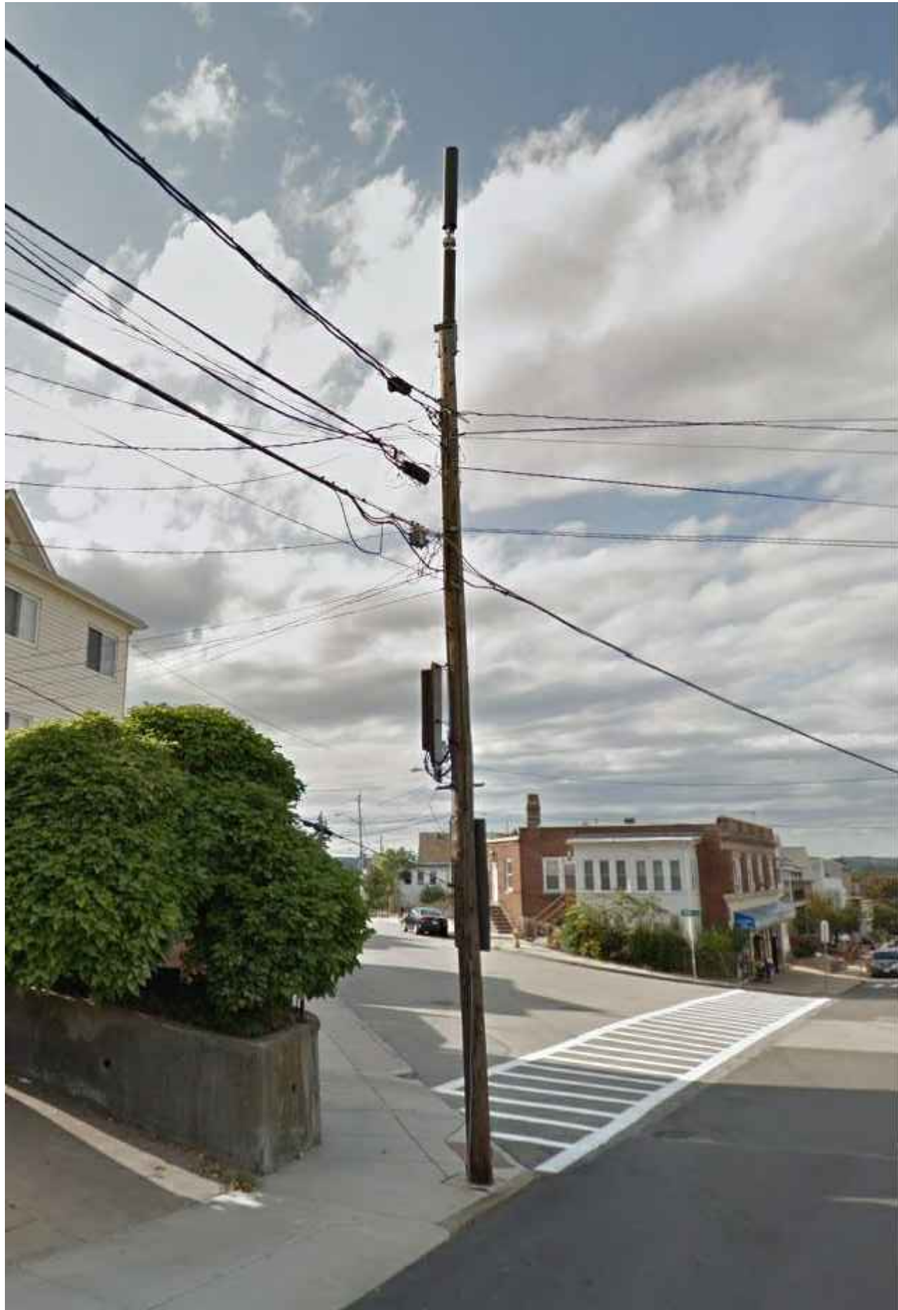
UTILITY POLE – BEFORE
