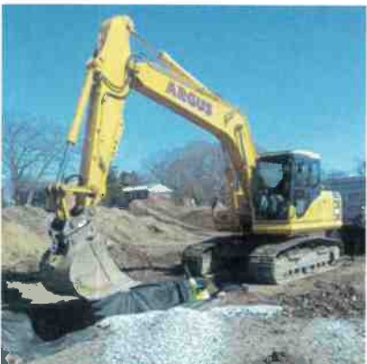
Construction, Almont Park - Mattapan
