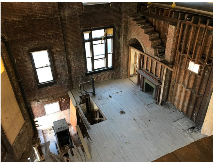
Interior of West Branch Library, currently under renovation
