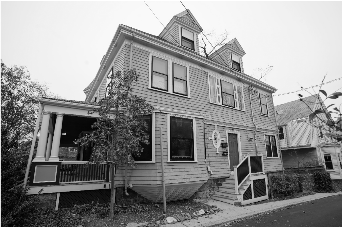
Photo 2 (E-1). South Elevation.
