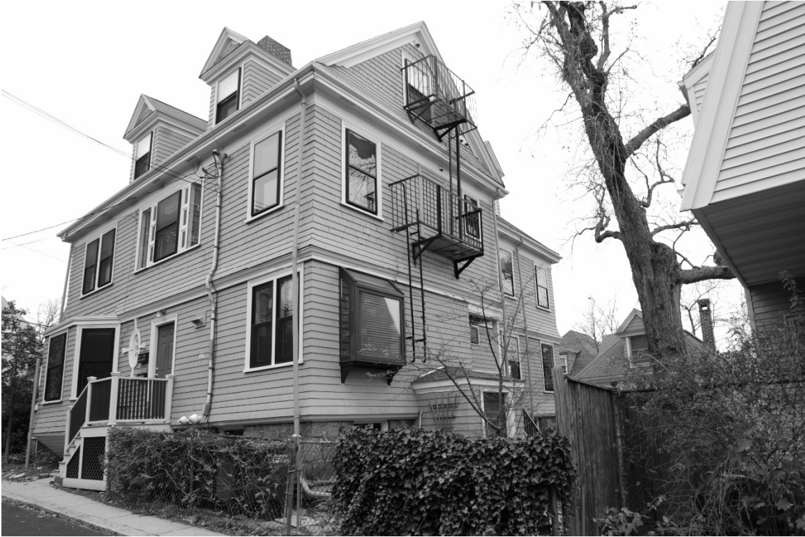
Photo 3 (E-1). South and East Elevations.
