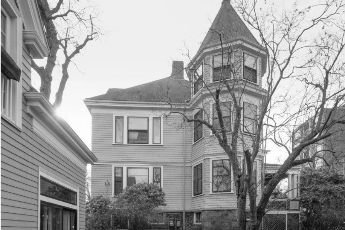
Photo 4 (E-1). North Elevation.
