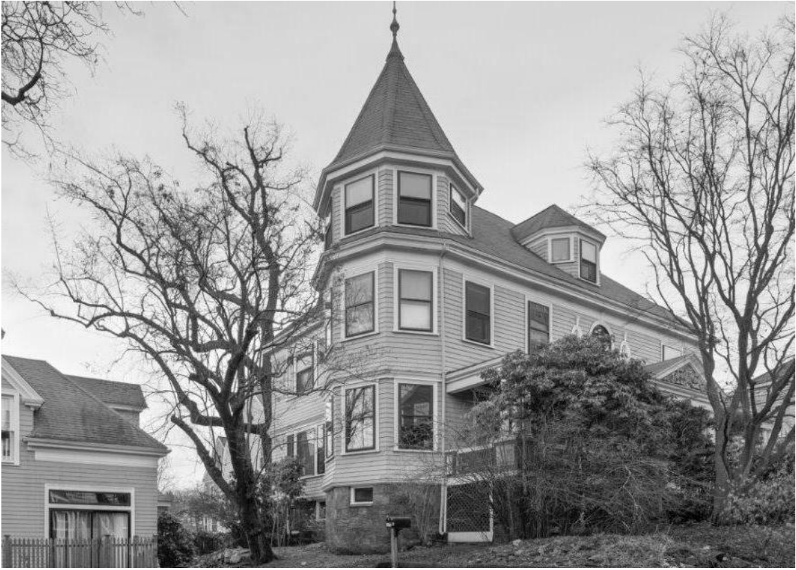
Photo 5. North and West Elevations.
