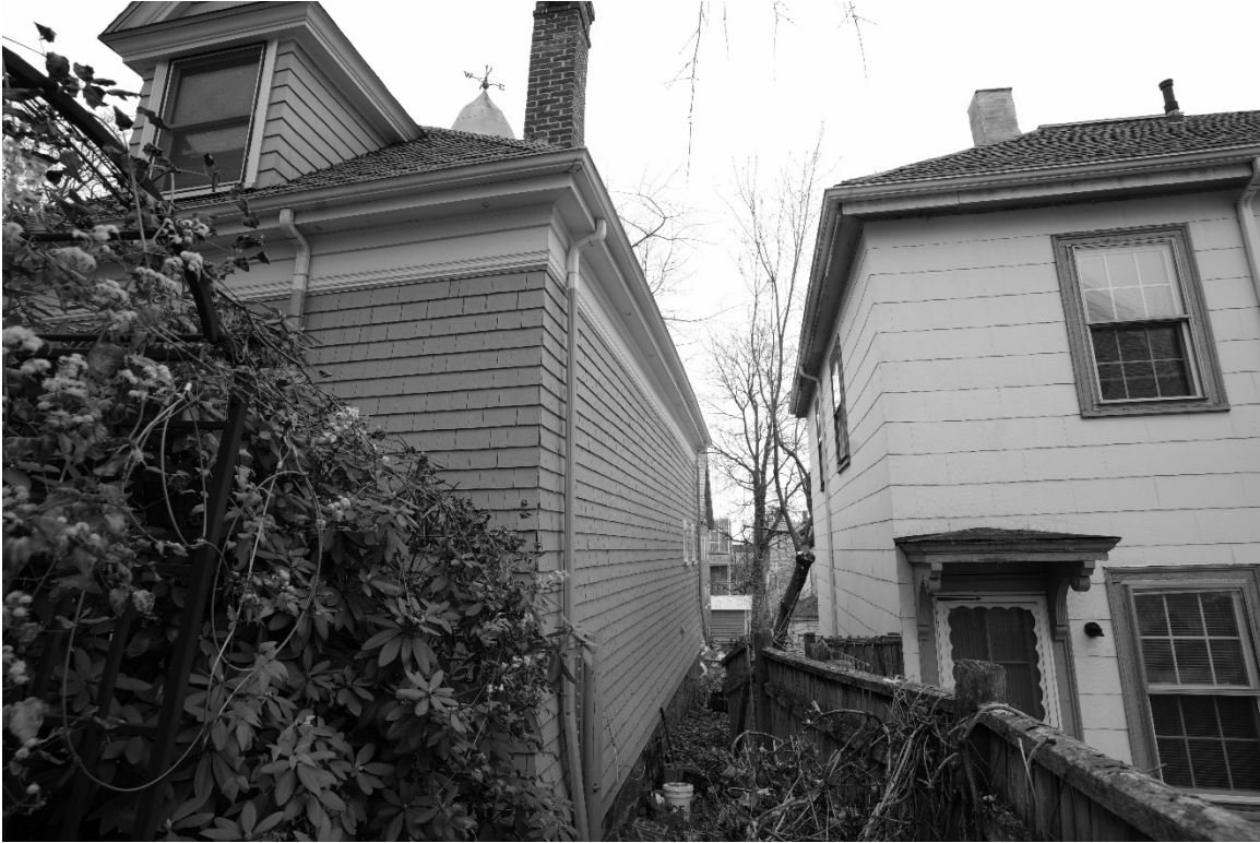
Photo 3. North and East Elevations.
