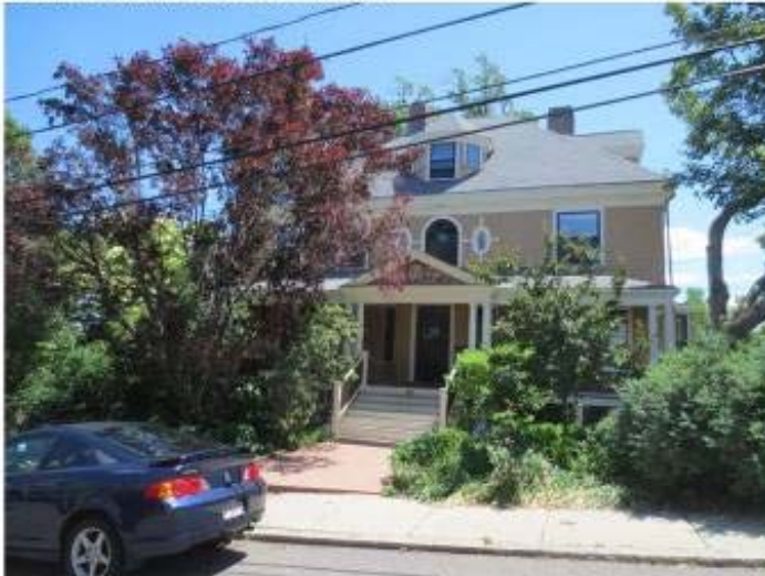
West elevation / façade of 83 Belmont Street
