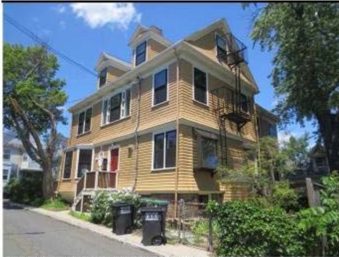
South and East elevations of 83 Belmont Street
