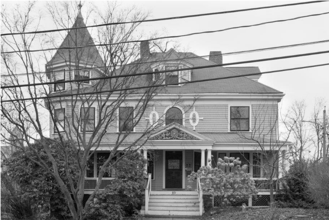
Photo 1 (E-1). West Elevation.
