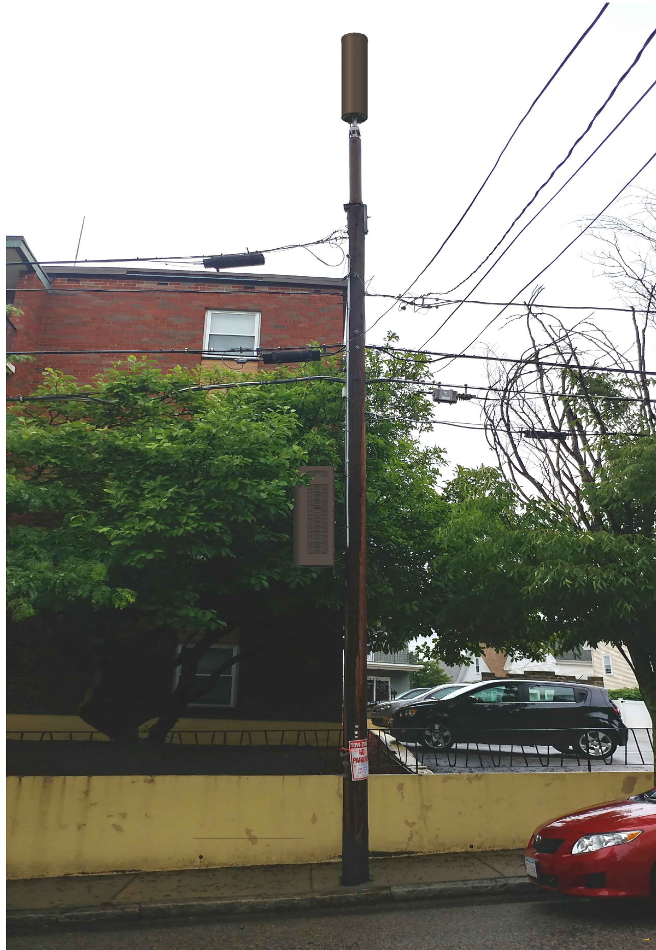
UTILITY POLE – AFTER
