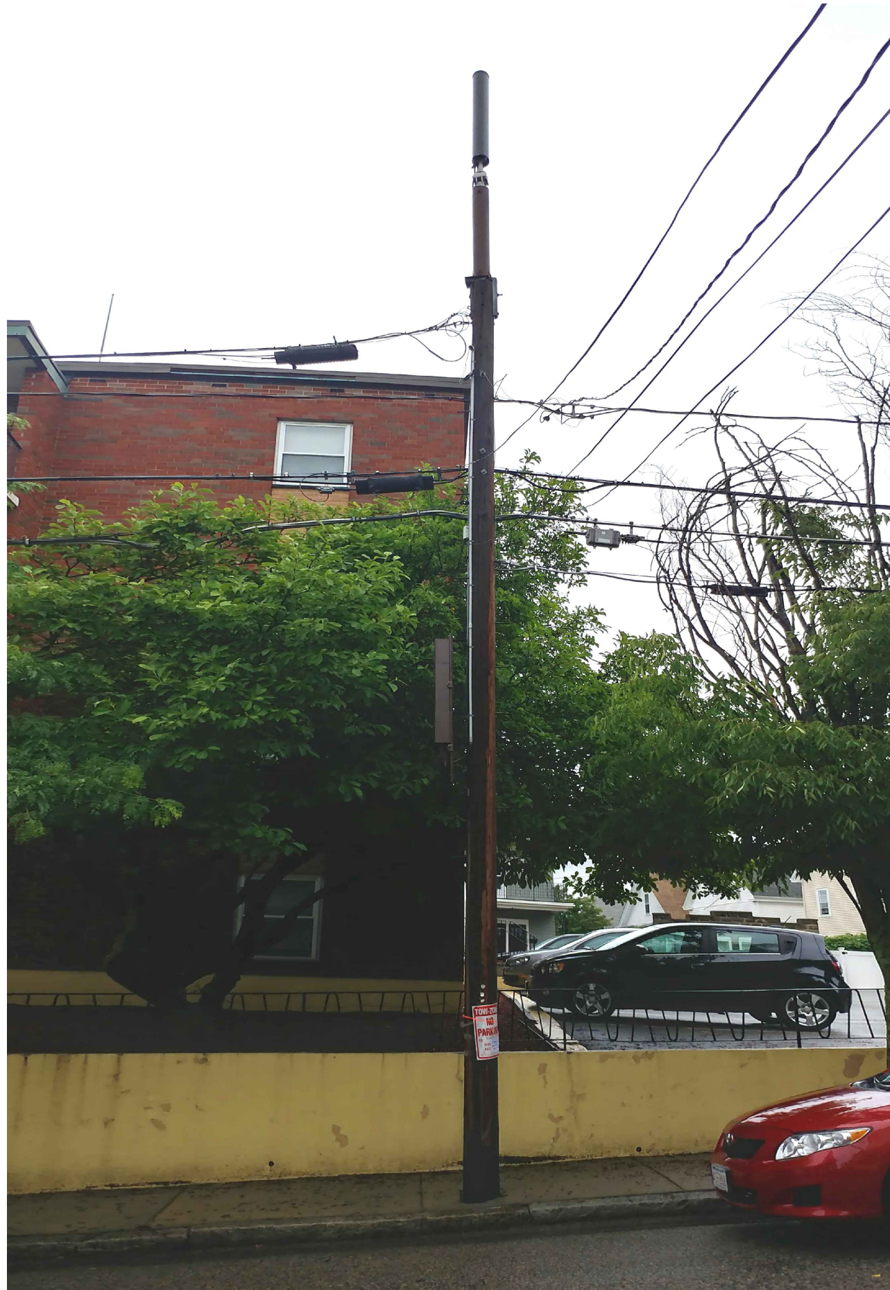
UTILITY POLE – BEFORE
