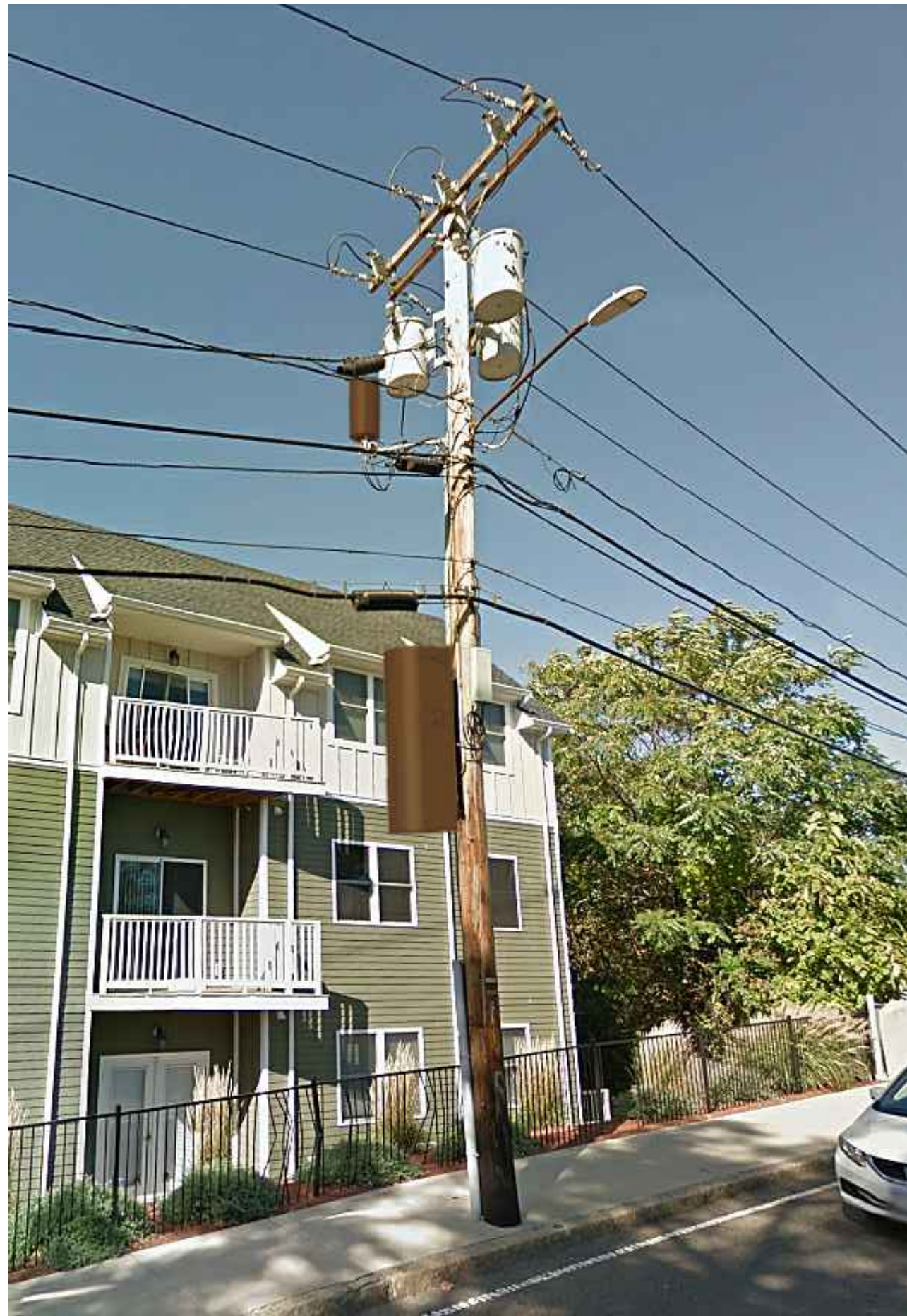
UTILITY POLE – AFTER
