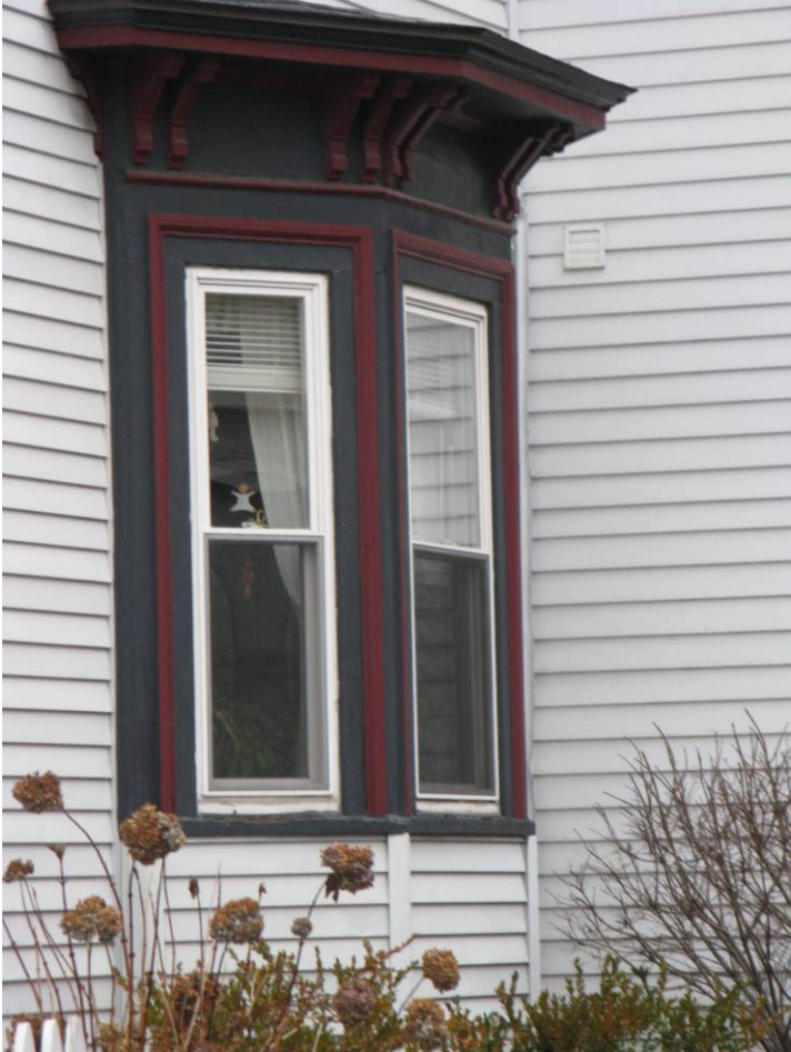
Detail of bay window with original sawn wood brackets
