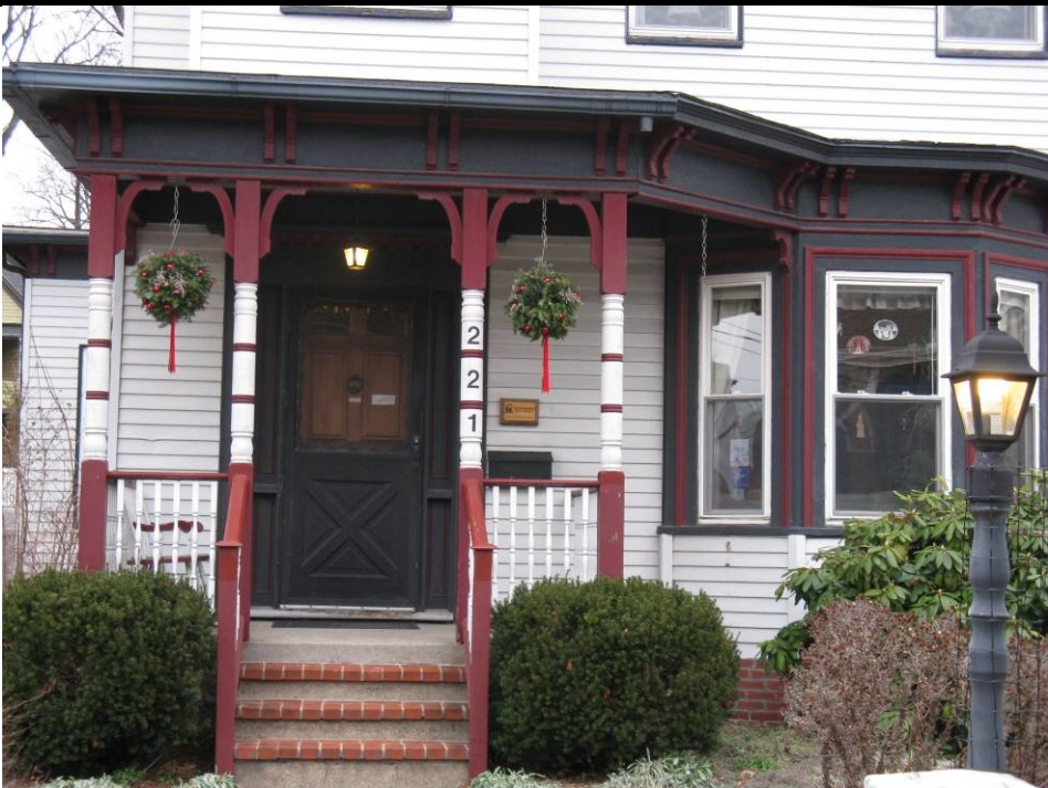
Detail of main entry with replicated sawn wood brackets.
