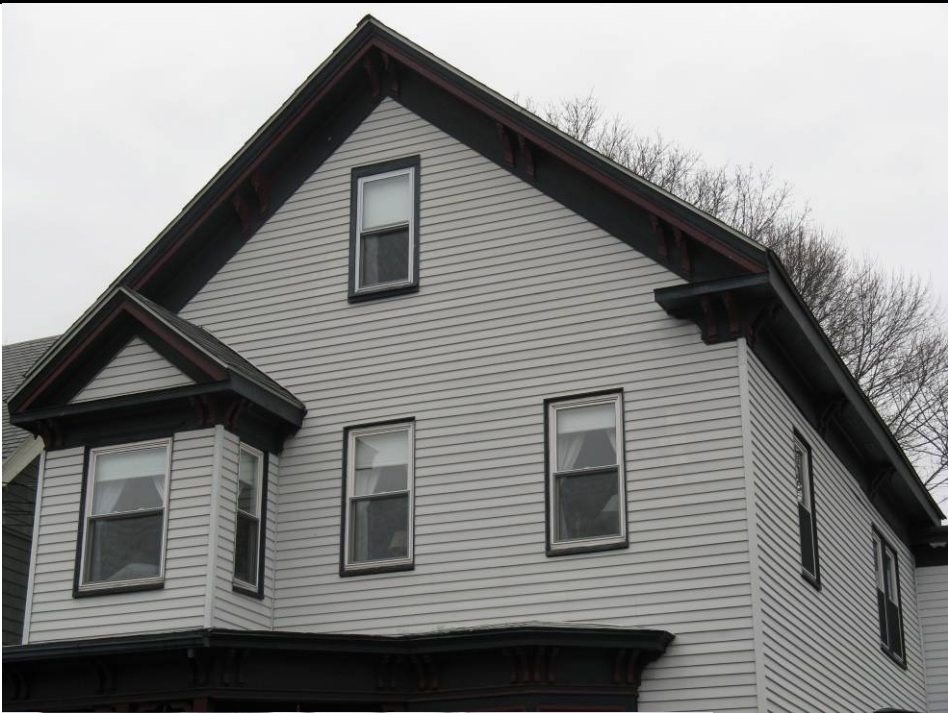
Roof line showing paired sawn wood brackets.
