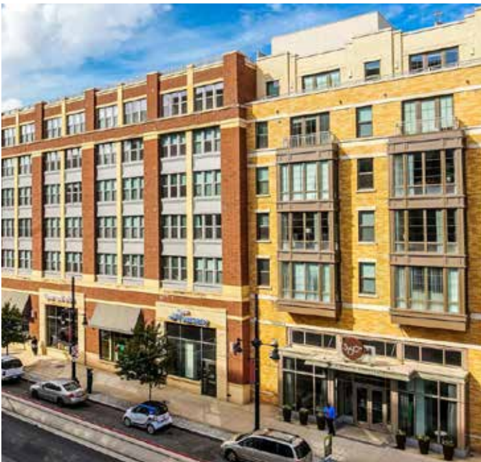
Figure 4.2.11 (b) Appearance of Two Buildings
