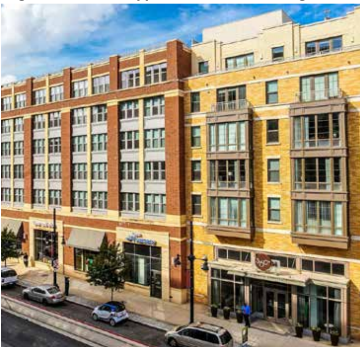
Figure 4.3.11 (b) Appearance of Two Buildings
