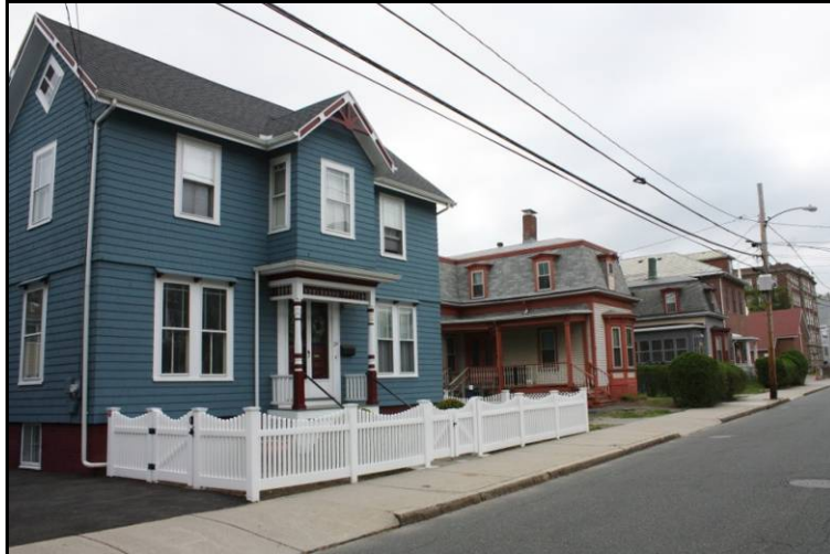
South side of Morrison Avenue: The first Mansard cottage is 222 Morrison Avenue, also included within the Morrison Avenue Local Historic District
