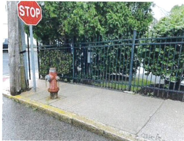
Lack of access from side street
