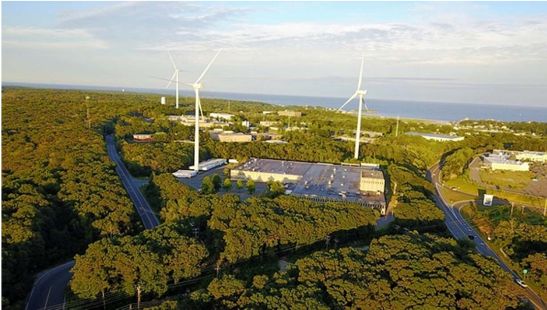
Green Municipal Aggregations in Massachusetts support the two 2-megawatt wind turbines in the foreground at Blackburn Industrial Park in Gloucester, MA
