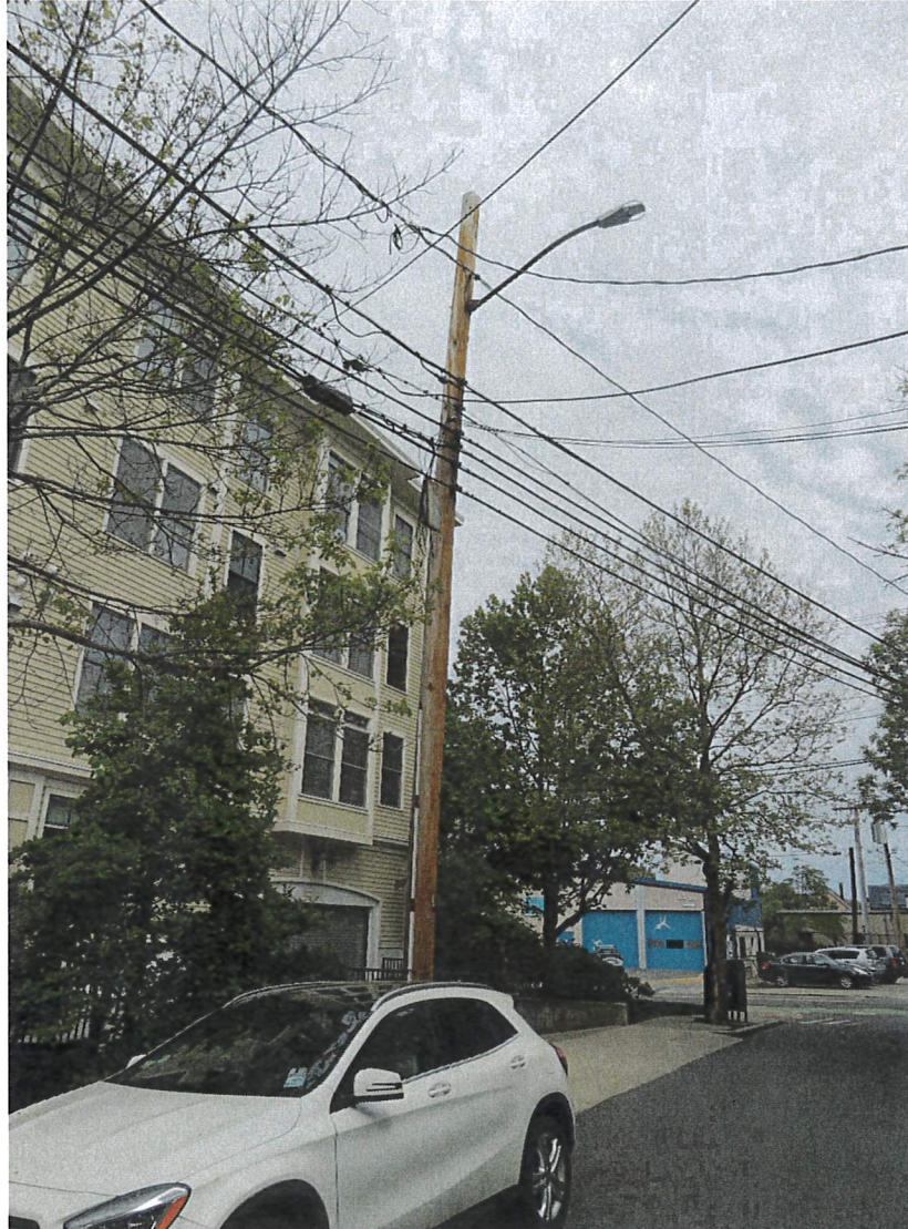
Photo 1: Sample photo illustrating the existing wood pole.
