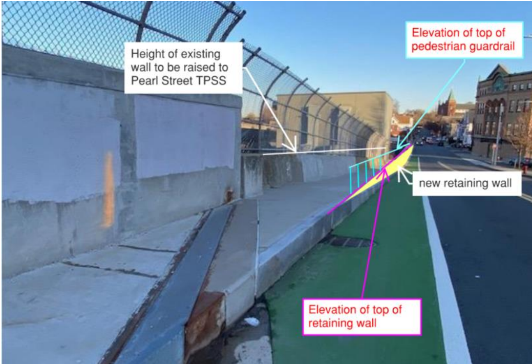
Figure 1: Medford Street looking North (from rail bridge)
