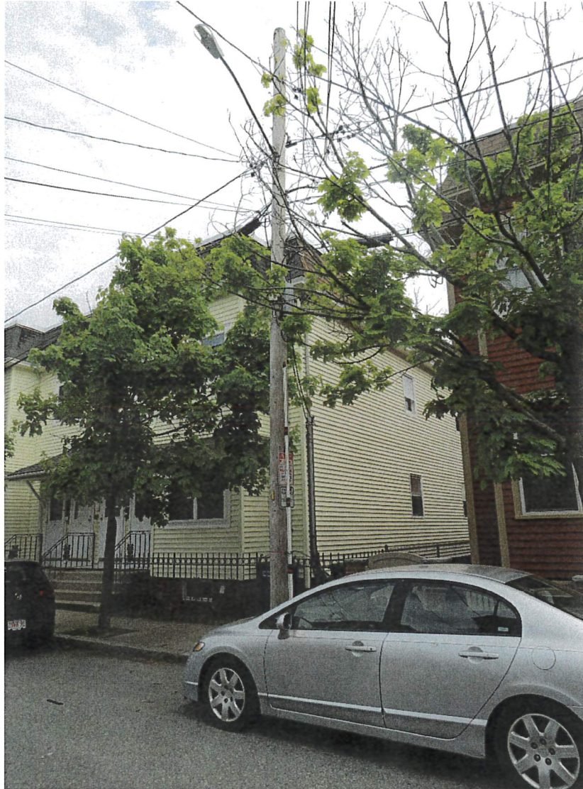
Photo 1: Sample photo illustrating the existing wood pole.
