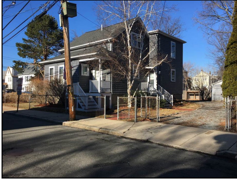
Right façade and garage for 31 Richardson
