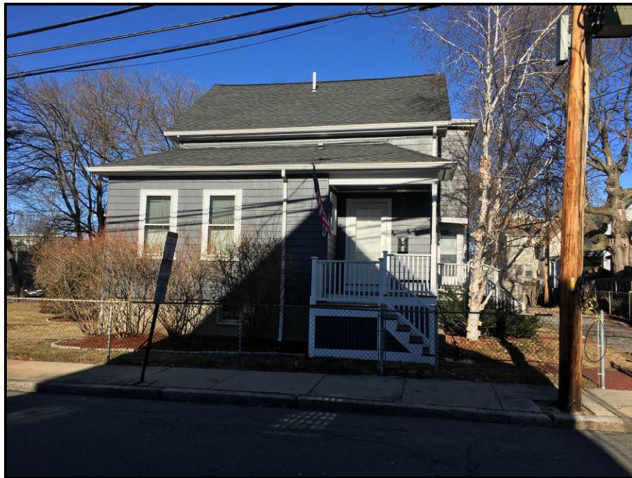
Richardson Street façade of 31 Richardson
