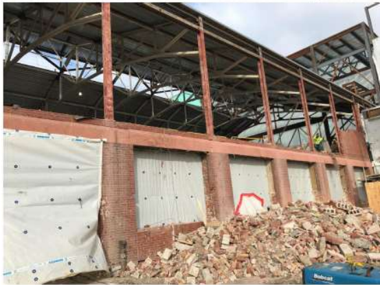
War Memorial Building ( January 2020 ) Post-demolition discovery of structural issues, requiring full facade demolition and structural repairs.
