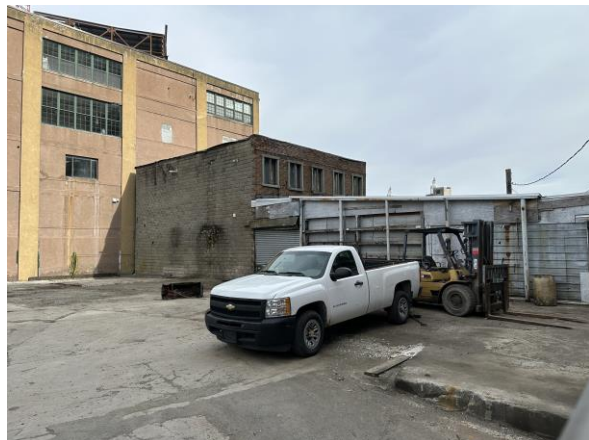
Looking south at subject
