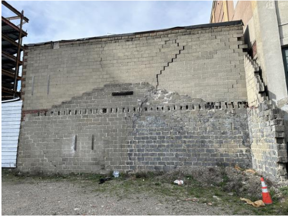
Looking north at subject exterior from adjacent property
