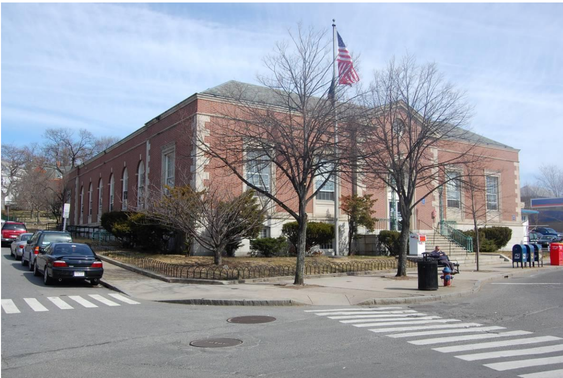
Photograph 2. View of facade and west elevations looking northeast from Washington Street.
