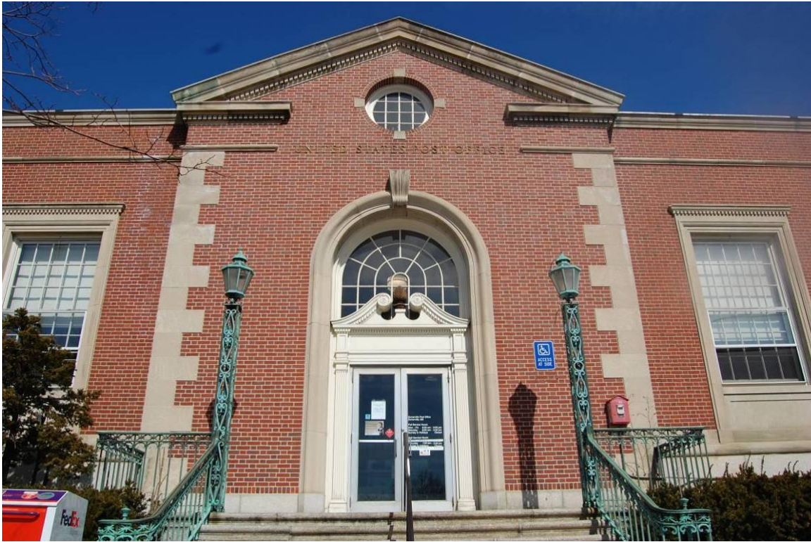
Photograph 5. Detail of main entrance.
