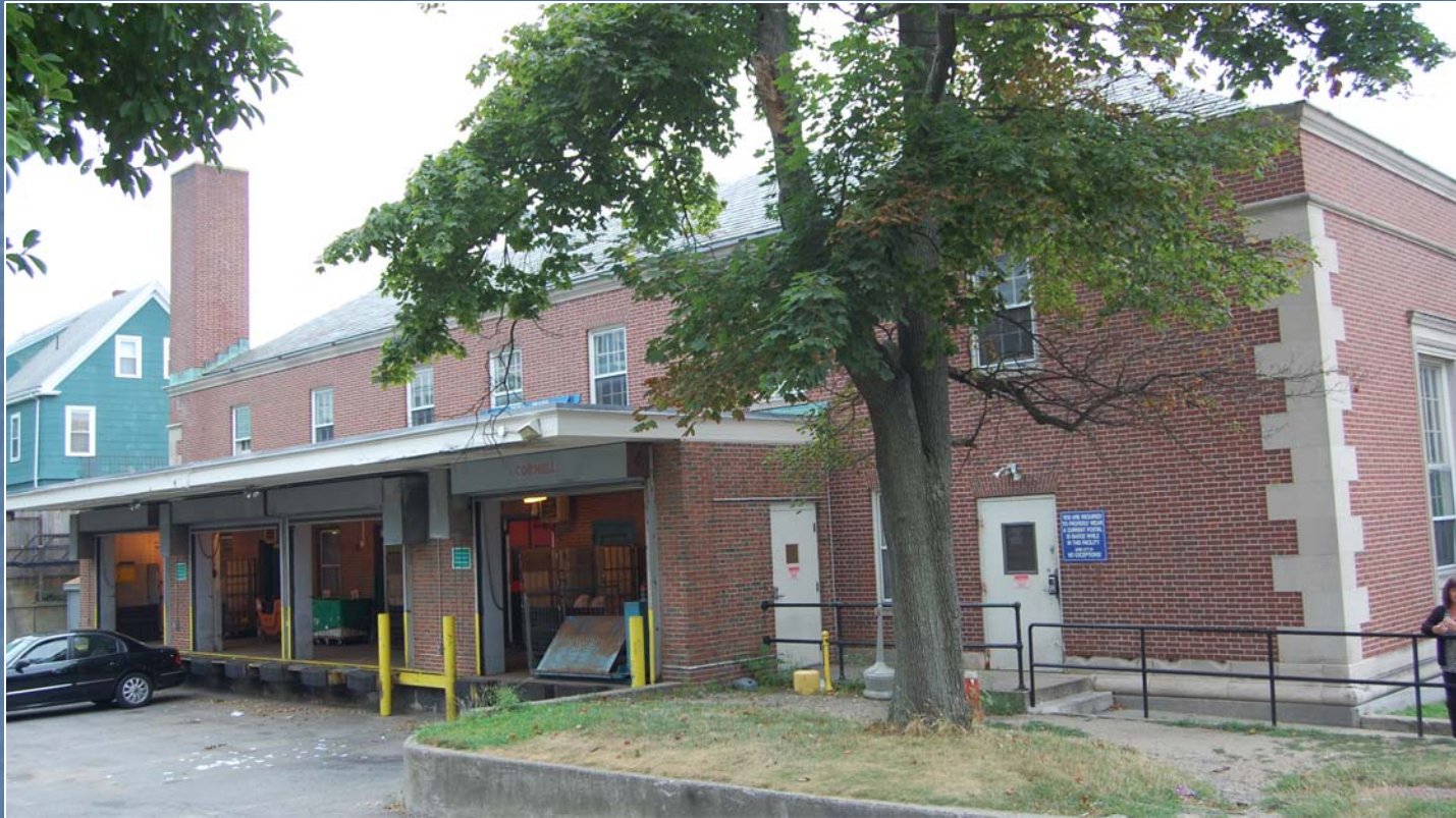
Rear elevation looking southeast from Bonner Avenue
