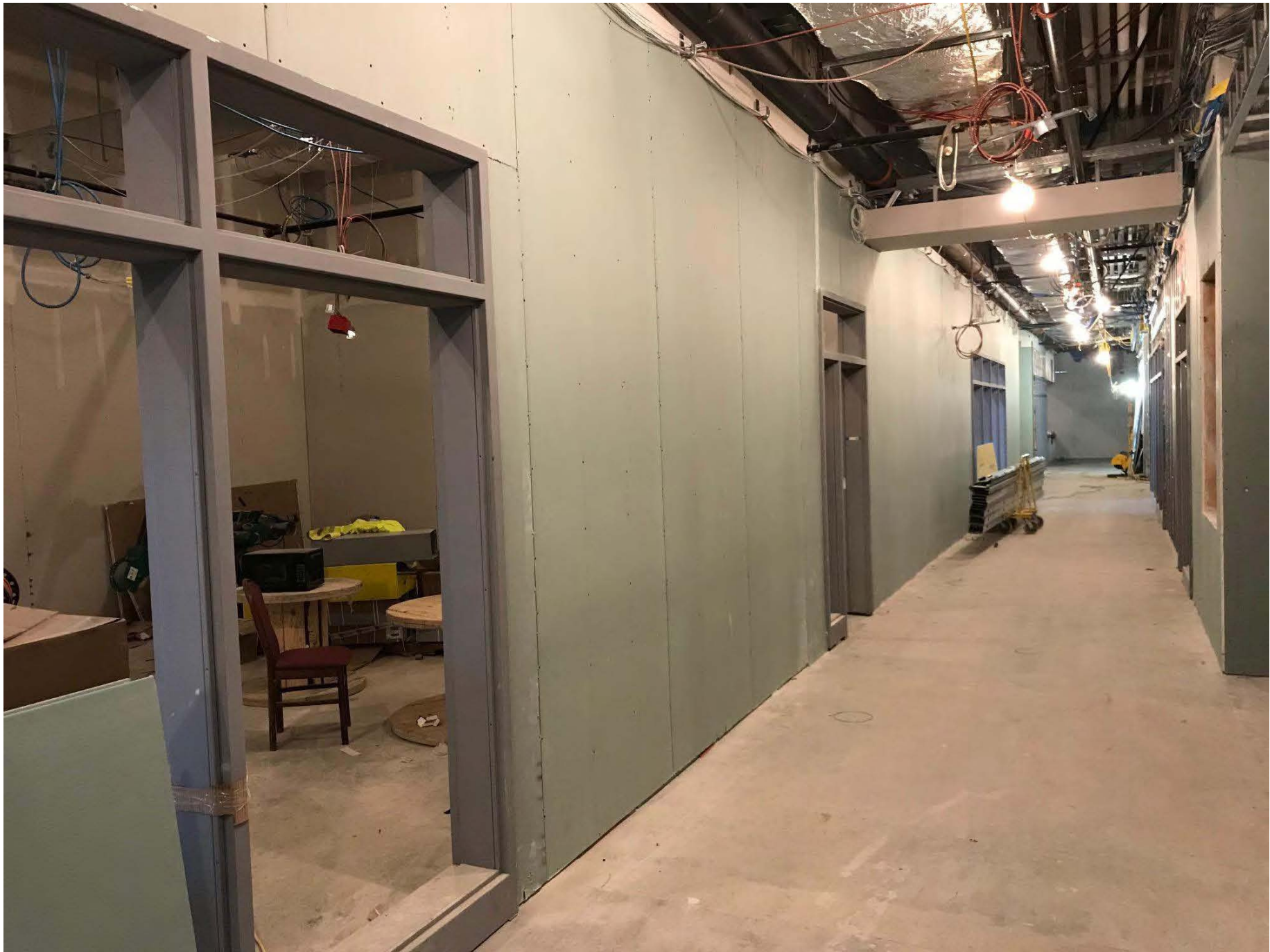
Phase 1A (Field House Lower Level) - Drywall (Closing Walls) January 2020
