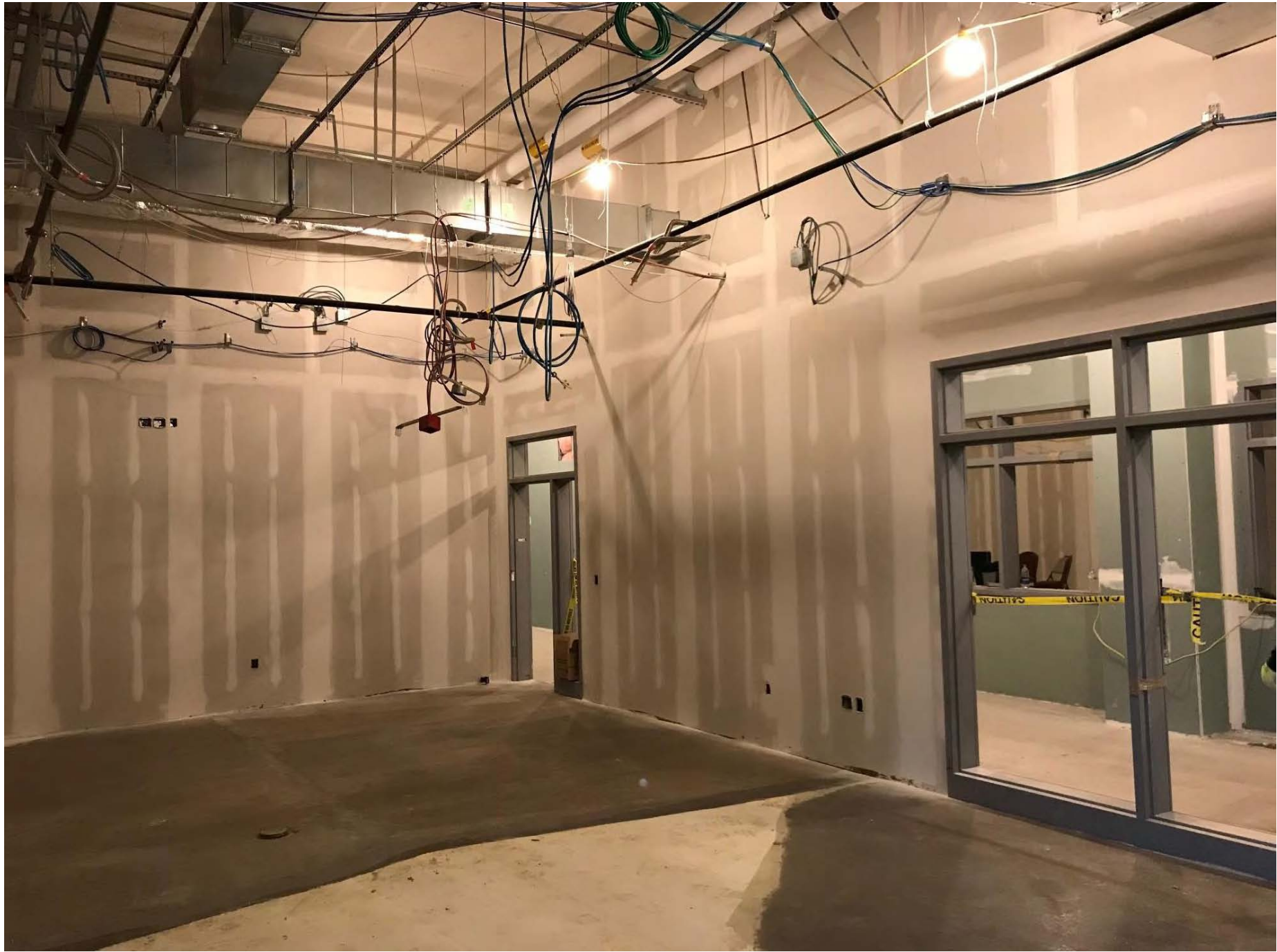
Phase 1A (Field House Lower Level) - Drywall (Taping, Near Ready for Paint) February 2020
