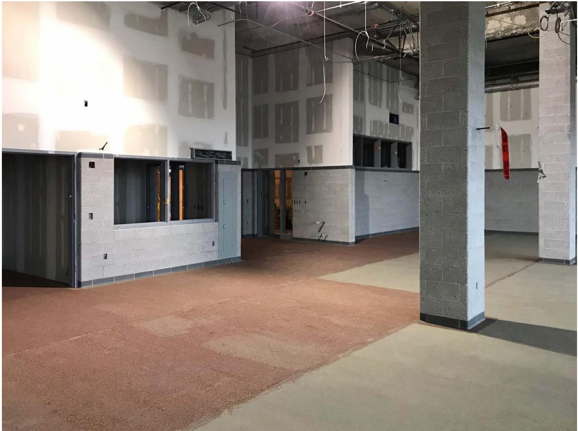
Phase 1A - CMU Walls / Drywall Taping February 2020
