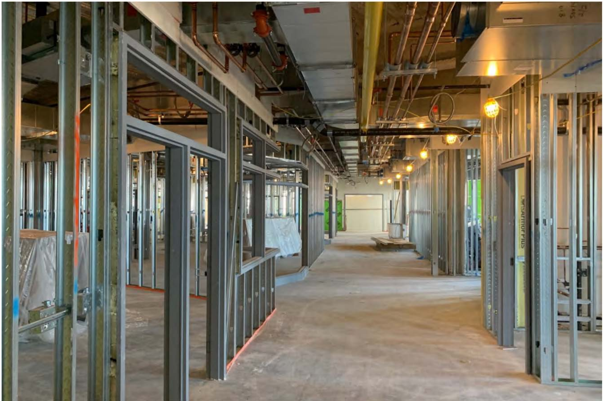
Phase 2 MEP Rough-in / Framing April 2020
