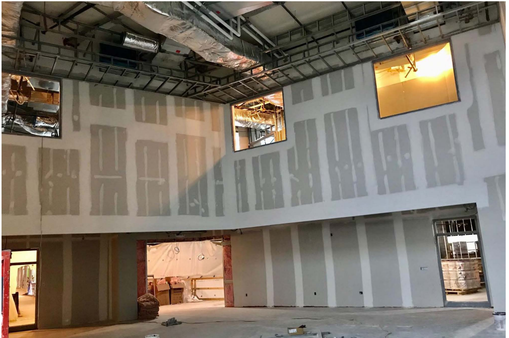
Phase 1 - Level 2 / Orchestra Room (GWB / Tape, Nearing Ready for Paint) February 2020
