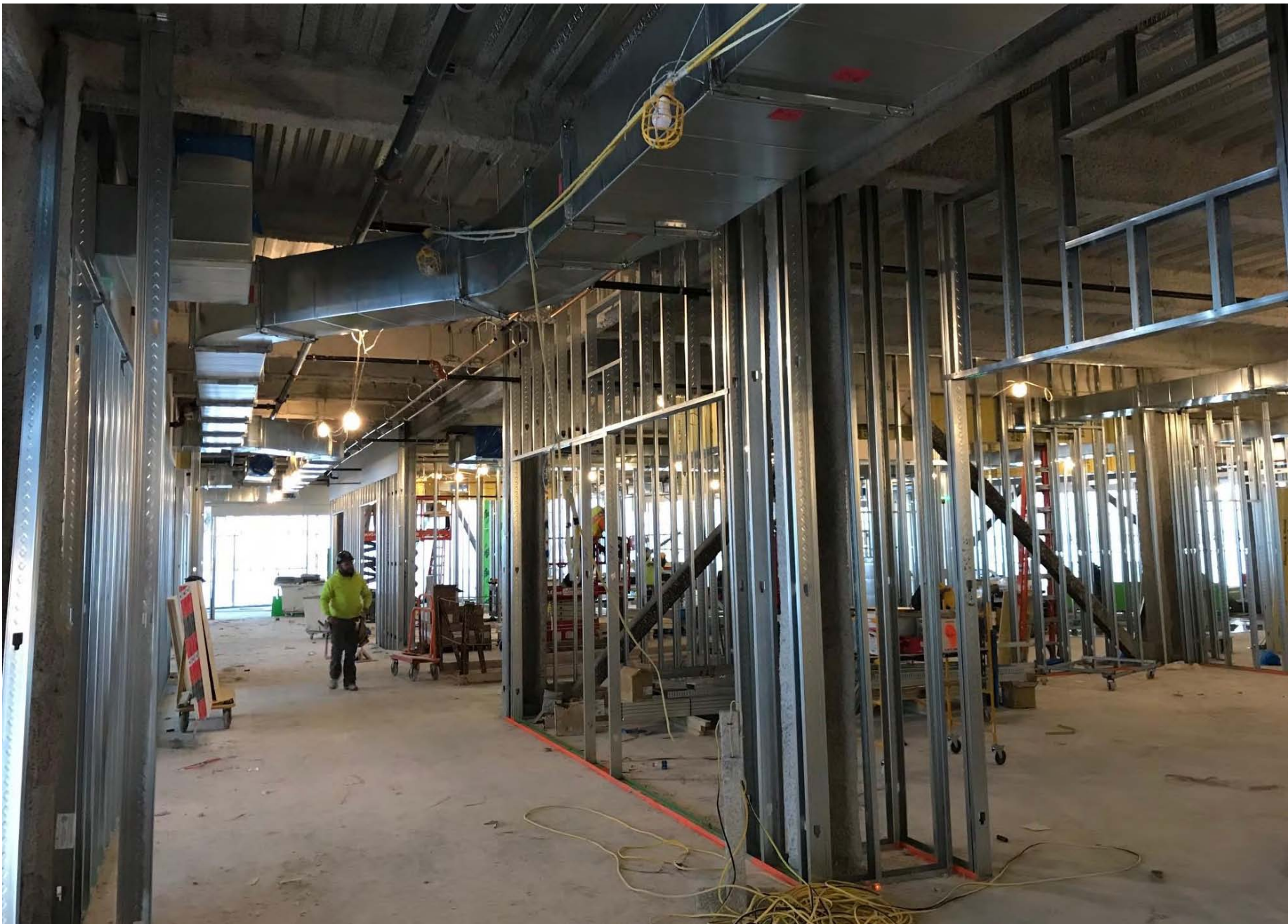
Phase 2 - Level 2 MEP Overhead Rough-in, Drywall Framing February 2020
