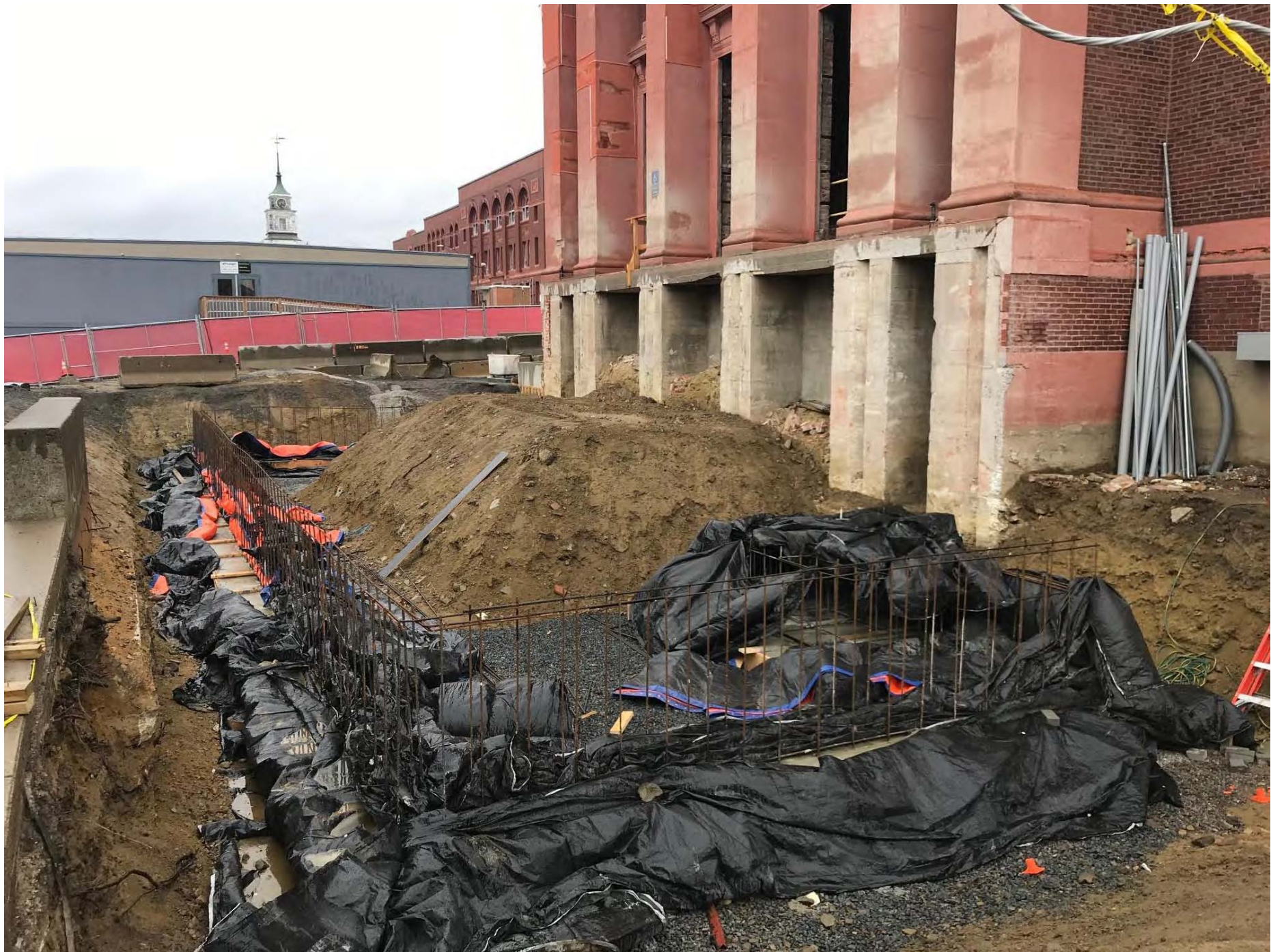
Phase 2A - Excavation and Footings for New Monumental Stairs February 2020
