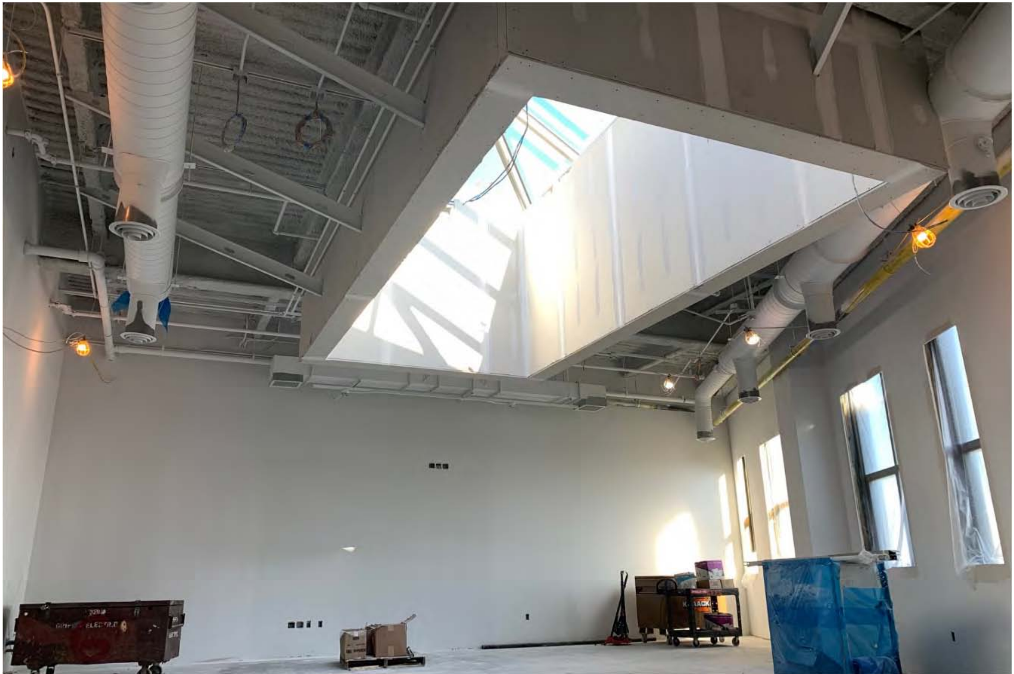
Phase 1 - Level 4 Mechanical Rough-in Complete, Ready for Ceilings / Flooring April 2020
