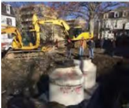
This page: Stormwater retention chambers were included in the redesign of both Symphony and Lincoln Park.
