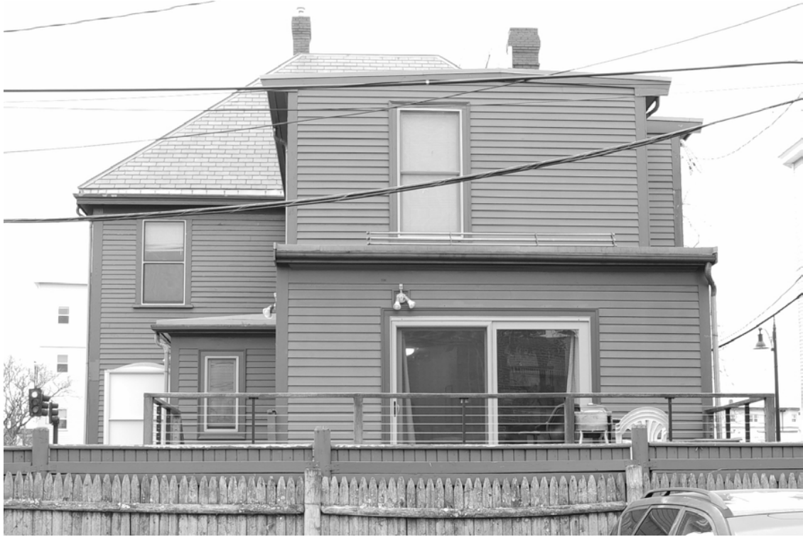
Photo 5. View of rear (northeast) elevations, looking southwest.
