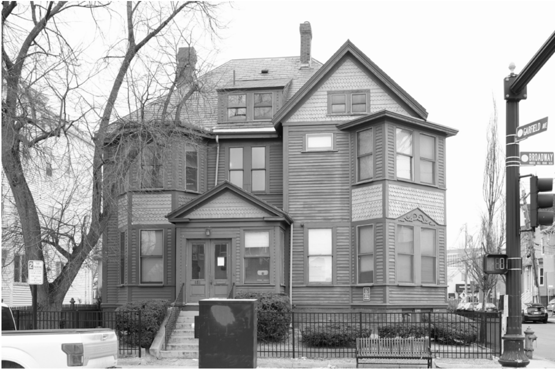
Photo 1. View of front (southwest) elevation, looking northeast.
