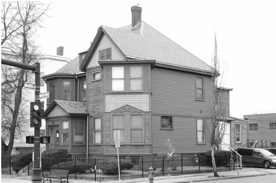
Photo 2. View of front (southwest) and right (southeast) side elevations, looking north.
