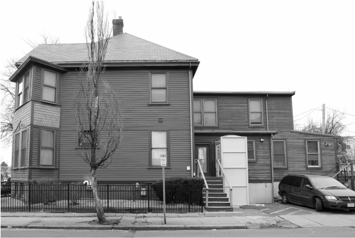
Photo 3. View of right (southeast) side elevations, looking northwest.
