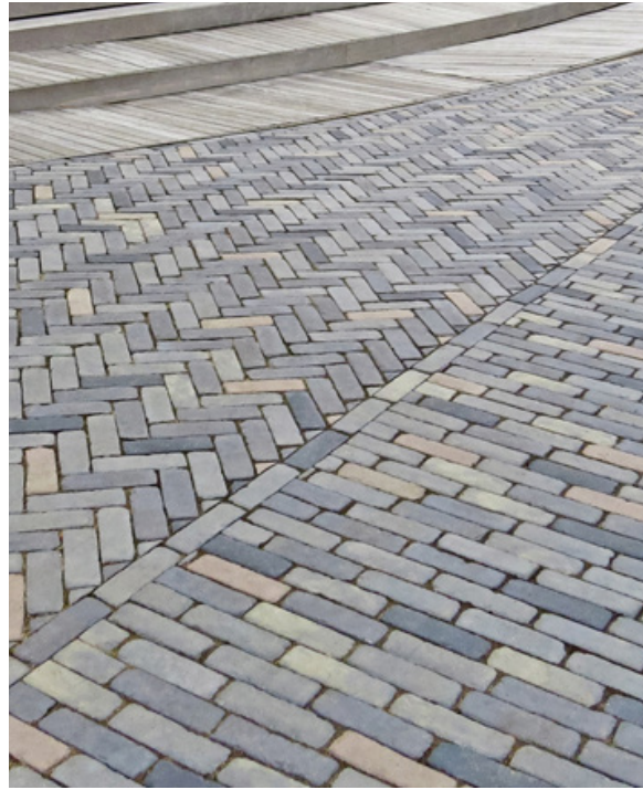
Small Format Permeable Pavers
