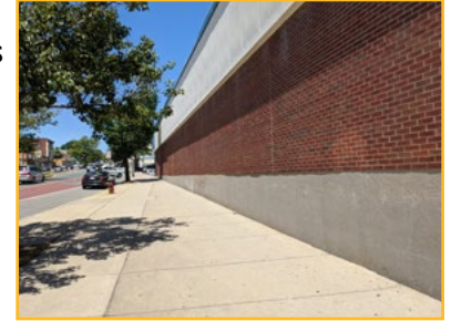
The pedestrian experience alongside the Project Area.
