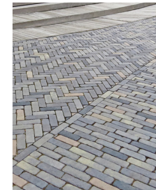
Small Format Permeable Pavers
