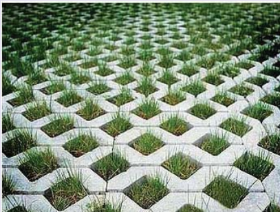
Pervious pavers use materials that allow water to percolate through.
