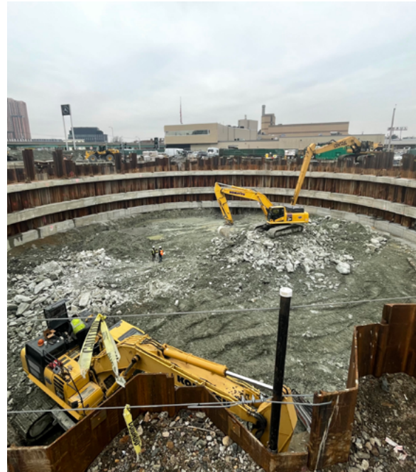
Excavation at the site of the Poplar Pump Station for future stormwater storage.
