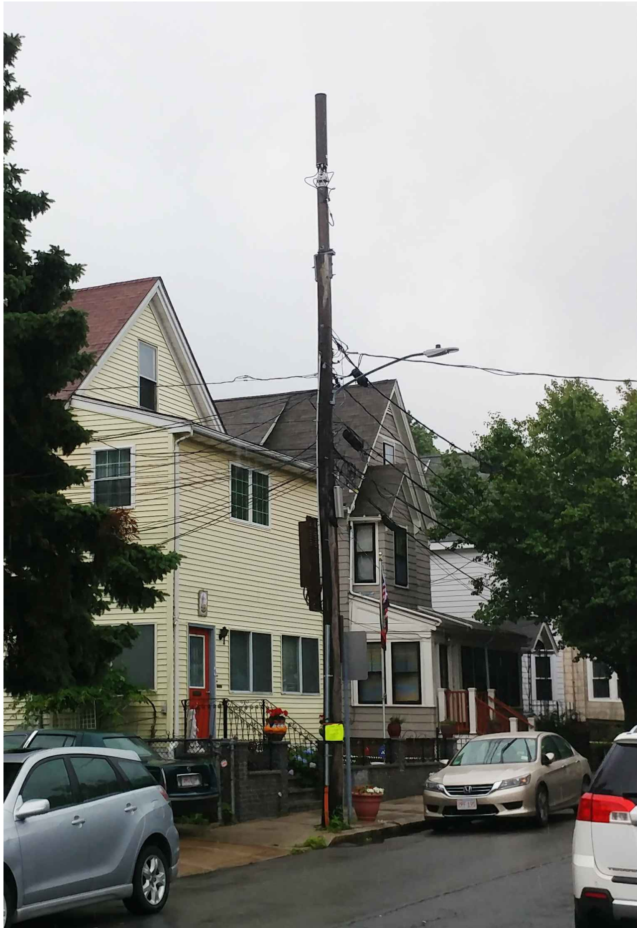
UTILITY POLE – BEFORE
