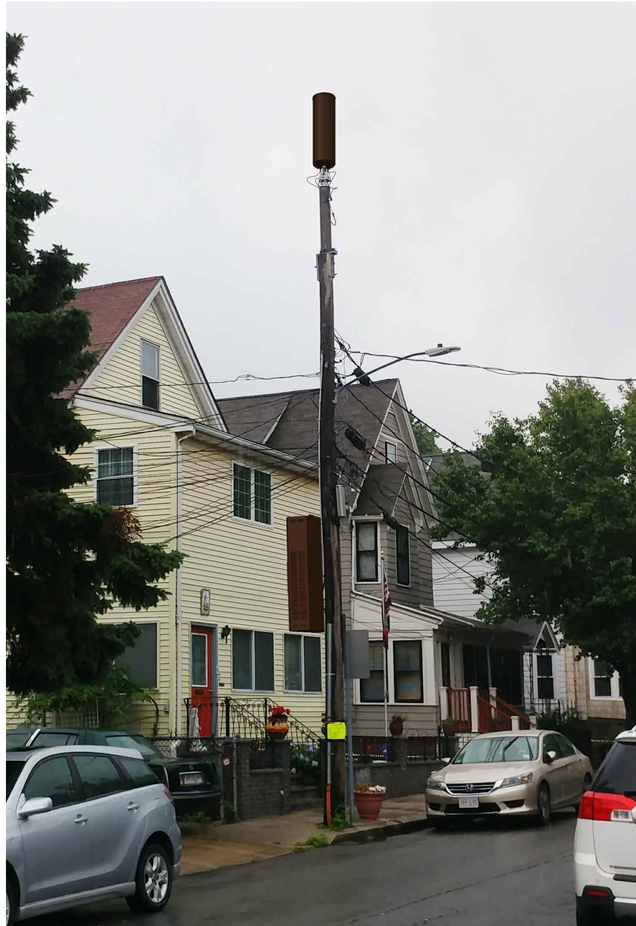
UTILITY POLE – AFTER
