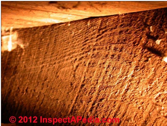
Figure 2 – Circular sawmill markings
