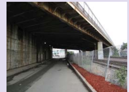
Current connection under McGrath Highway at Somerville Avenue
