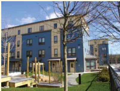
Phase 2 of the Somerville Community Corporation's St. Polycarp's Village, completed in 2011, includes 29 units of purpose-built affordable housing.
