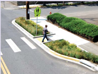
A bumpout makes visibility easier for pedestrians, drivers, and cyclists, adds green space, and shortens crossing lengths.
