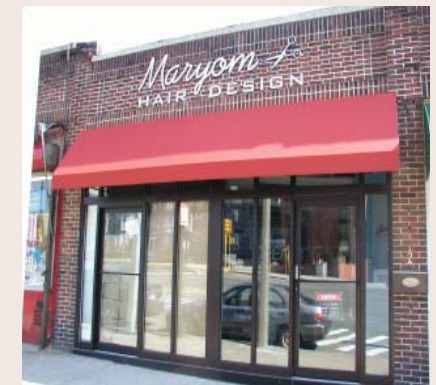
In 2009, Winter Hill's Maryom Hair Design used the City's Storefront Improvement Program to pay for facade improvements.
