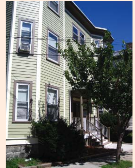
Two of the units at the Somerville Community Corporation's Gilman Street property are earmarked for formerly homeless households.
