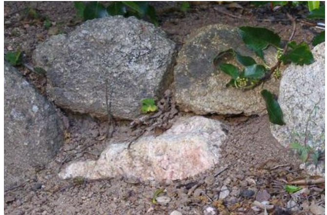
Dry stack walls are rocks stacked on each other.
