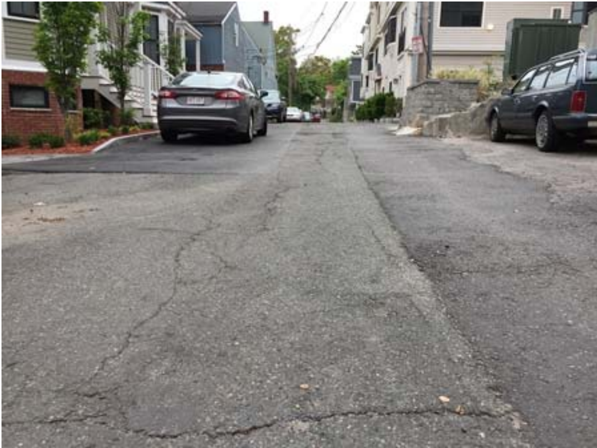
Figure 2 Gas Trenches on Either Side of Original Pavement
