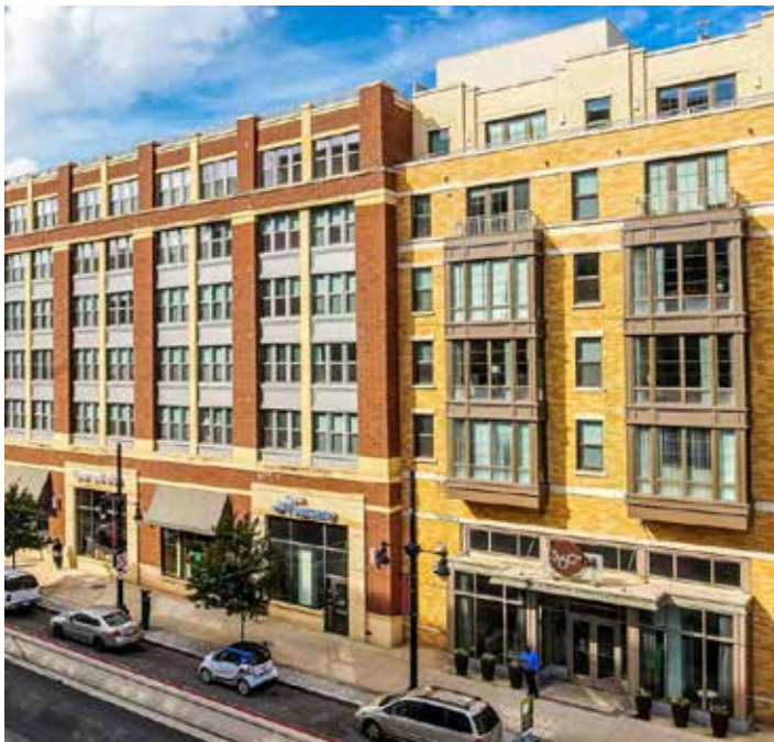
Figure 6.2.9 Appearance of Two Buildings
