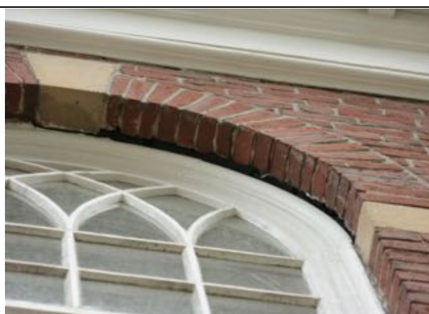
Gap between wood window frame and adjacent brickwork: Round-arched window on south elevation.
