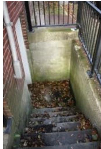
Areaway at northeast corner of building: Accumulation of debris on landing and algae on walls.
