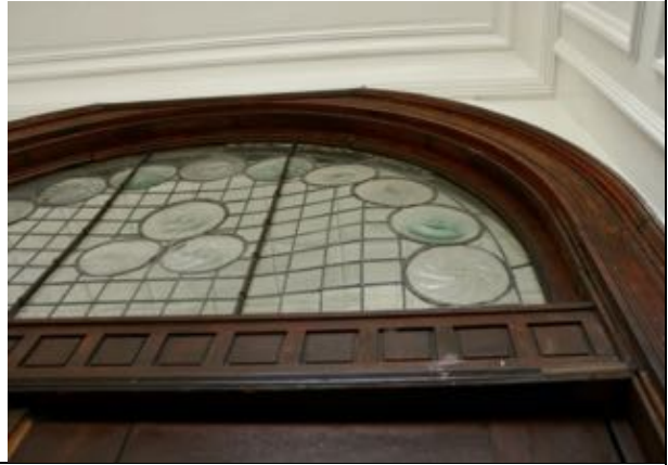
Leaded glass transom in entry foyer adjacent to Main Gallery: Buckled glass at north end.
