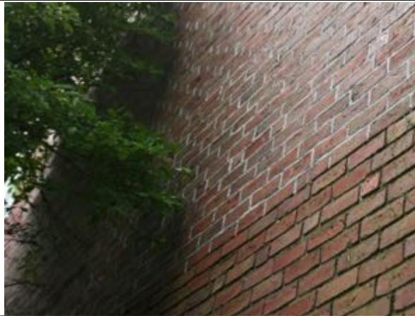
North elevation: Mortar erosion at bottom half of wall.
