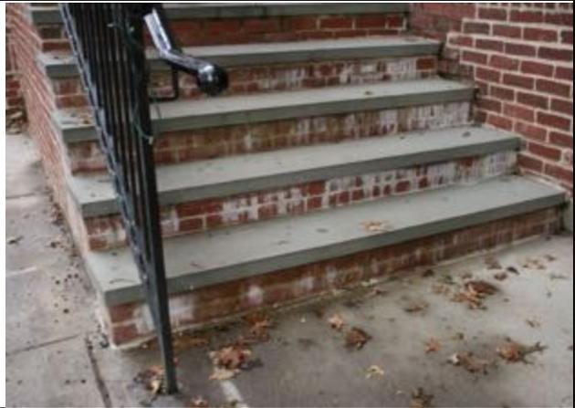
South elevation: Efflorescence on entry stairway.
