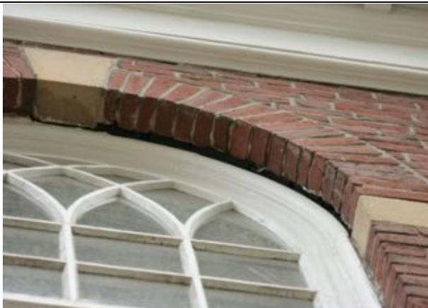
Gap between wood window frame and adjacent brickwork: Round-arched window on south elevation.
