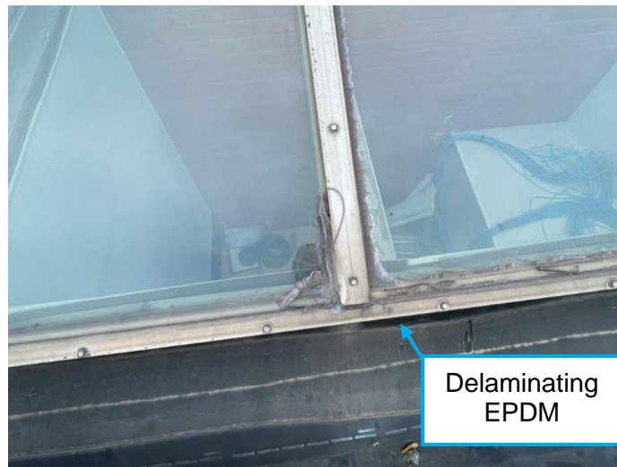
Photo 5 – Sloped skylight at West elevation. EPDM membrane is delaminating at skylight curb.
