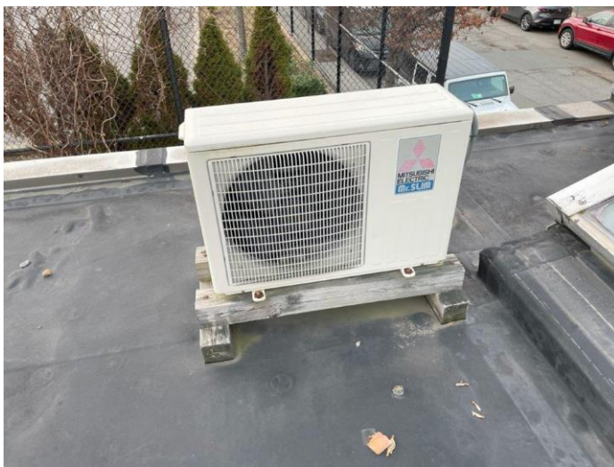
Photo 13 – Mitsubishi heat pump serving Electrical/IT Room.
