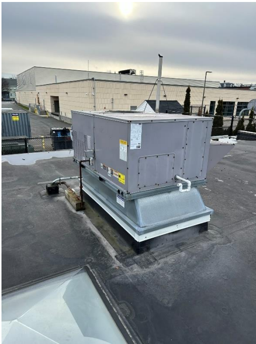
Photo 15– Carrier RTU 2. Blower door test showed 460 CFM air leakage at both RTUs when tested @-50Pa. Refer to Appendix D.
