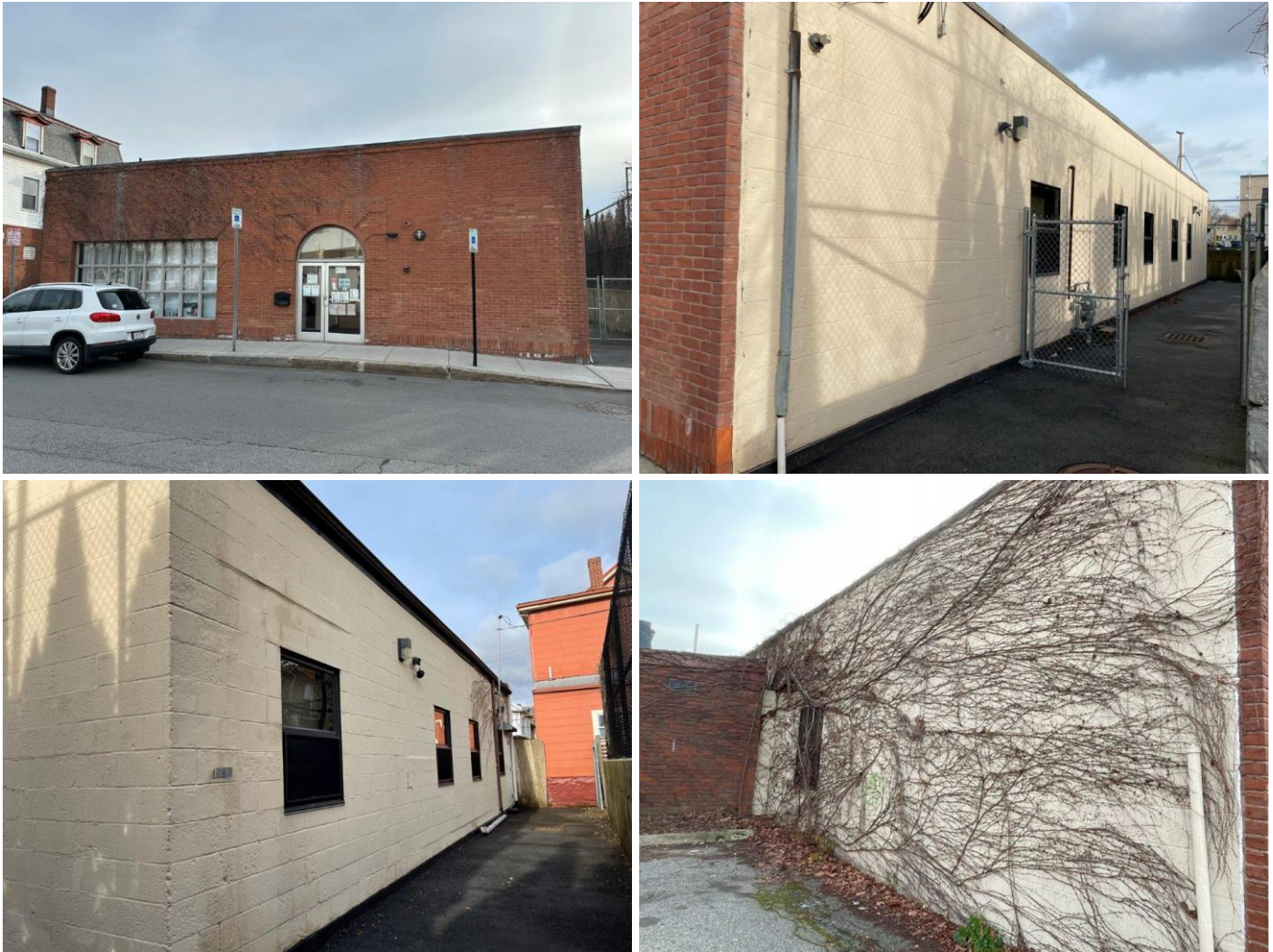
Photo 1 - West (top-left), South (top-right), East (bottom-left), and North (bottom-right) building elevations. Triple-wythe brick masonry wall on West elevation, and single-wythe CMU construction on other elevations. Vines need to be removed prior to roof replacement for roof edge access.
