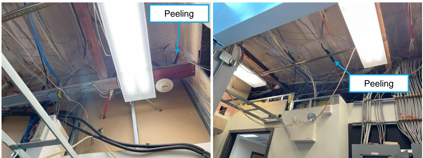
Photo 6 - Spray-foam insulation installed at underside of roof deck, as shown in the Electrical/IT room, is peeling and not continuous.
