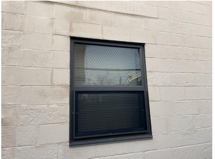
Photo 11 - Typical Winco window opening in open office area, installed in 2017. Blower door test showed 35 CFM air leakage across all punched windows (except for the windows located behind the archives storage, which remained sealed) when tested @-50Pa. Refer to Appendix D.
