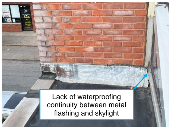
Photo 4 - Metal flashing at parapet. Low flashing height. Rough edges of flashing are touching the roof, which may cause punctures in the EPDM membrane. Flashing is not tied into skylight, relying only on sealant, and creating potential for water penetration at corner joint.
