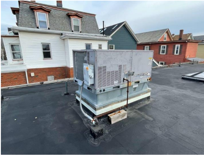
Photo 14– Carrier RTU 2. Blower door test showed 460 CFM air leakage at both RTUs when tested @-50Pa. Refer to Appendix D.
