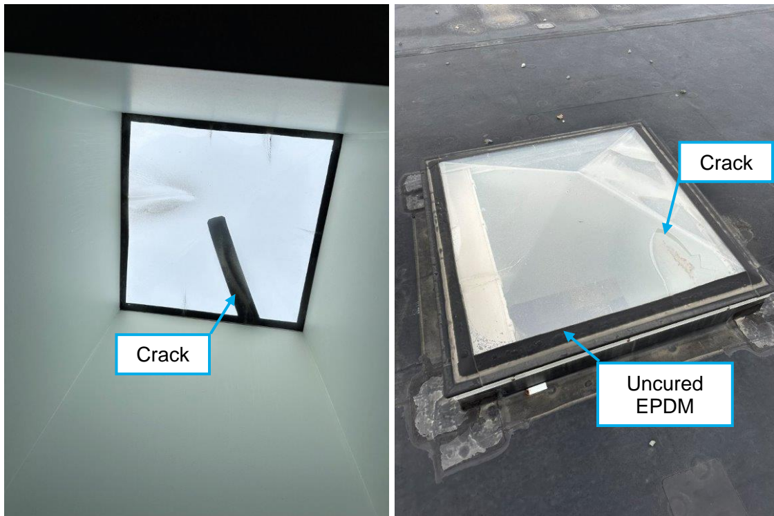
Photo 7 – Cracks in pyramid skylights. Uncured EPDM was installed at pyramid skylights, likely to stop leaking through the skylight at the metal frame/pyramid skylight interface. Blower door test showed 34 CFM air leakage when tested @-50Pa. Refer to Appendix D.
