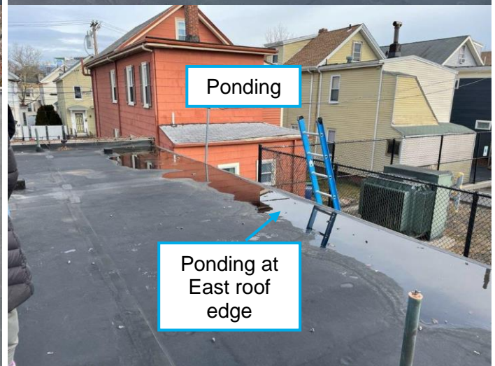
Photo 2 – Overview of Roof with Carlisle EPDM FR membrane. There is active ponding and residual dirt staining on the center of the roof, as well as areas of active ponding on the East roof edge. Rusted gooseneck penetrations should be wire-brushed and painted. The roof hatch has no interior access or exterior safety railing.
