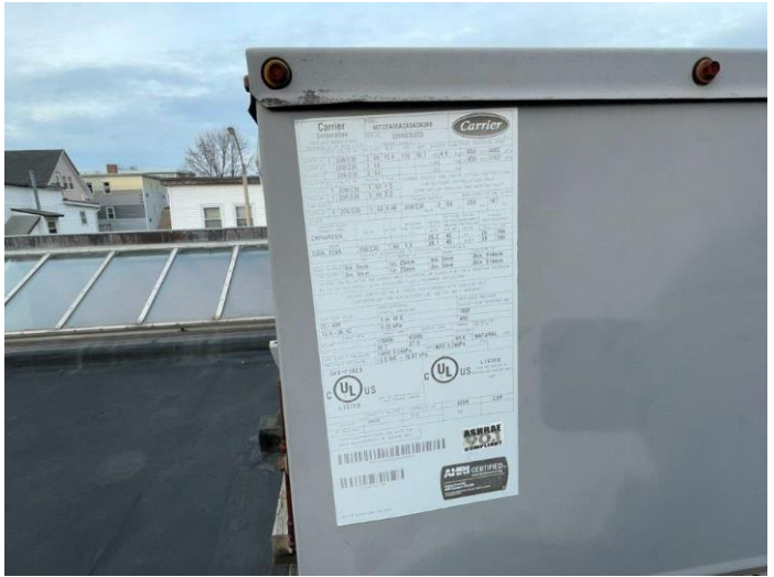
Photo 14– Carrier RTU 2. Blower door test showed 460 CFM air leakage at both RTUs when tested @-50Pa. Refer to Appendix D.
