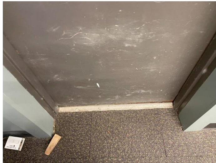
Photo 9 - Back egress door. Occupant seated near egress door has noted draftiness. Evidence of moisture damage is apparent at door head. Blower door test showed 123 CFM air leakage at egress door when tested at @-50Pa. Refer to Appendix D.
