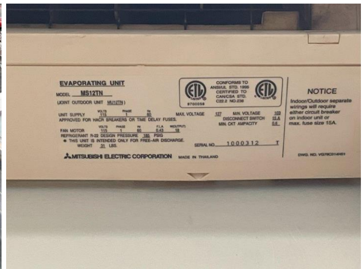
Photo 13 – Mitsubishi heat pump serving Electrical/IT Room.
