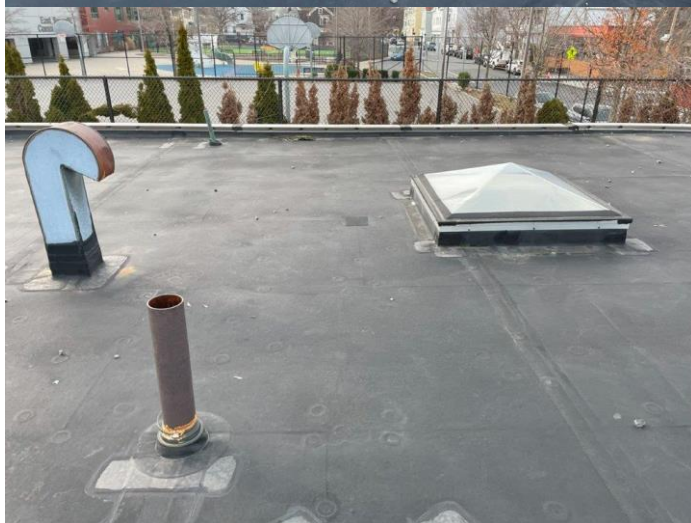
Photo 2 – Overview of Roof with Carlisle EPDM FR membrane. There is active ponding and residual dirt staining on the center of the roof, as well as areas of active ponding on the East roof edge. Rusted gooseneck penetrations should be wire-brushed and painted. The roof hatch has no interior access or exterior safety railing.
