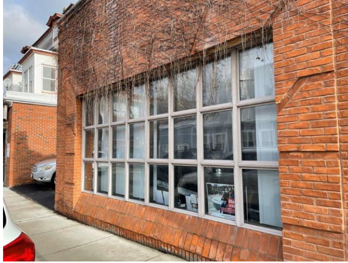
Photo 10 - Storefront window in Community Room. Blower door test showed 68 CFM air leakage at storefront when tested @-50Pa. Refer to Appendix D.
