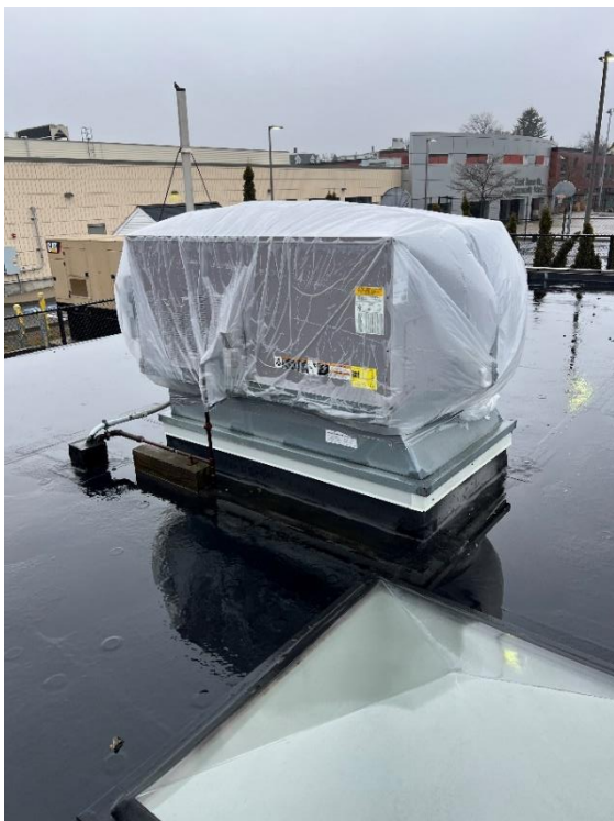
Photos 3-4: RTU Sealing
