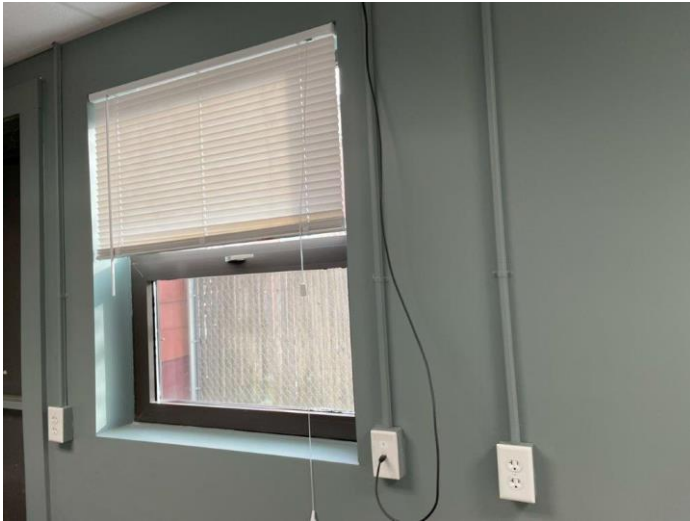
Photo 11 - Typical Winco window opening in open office area, installed in 2017. Blower door test showed 35 CFM air leakage across all punched windows (except for the windows located behind the archives storage, which remained sealed) when tested @-50Pa. Refer to Appendix D.
