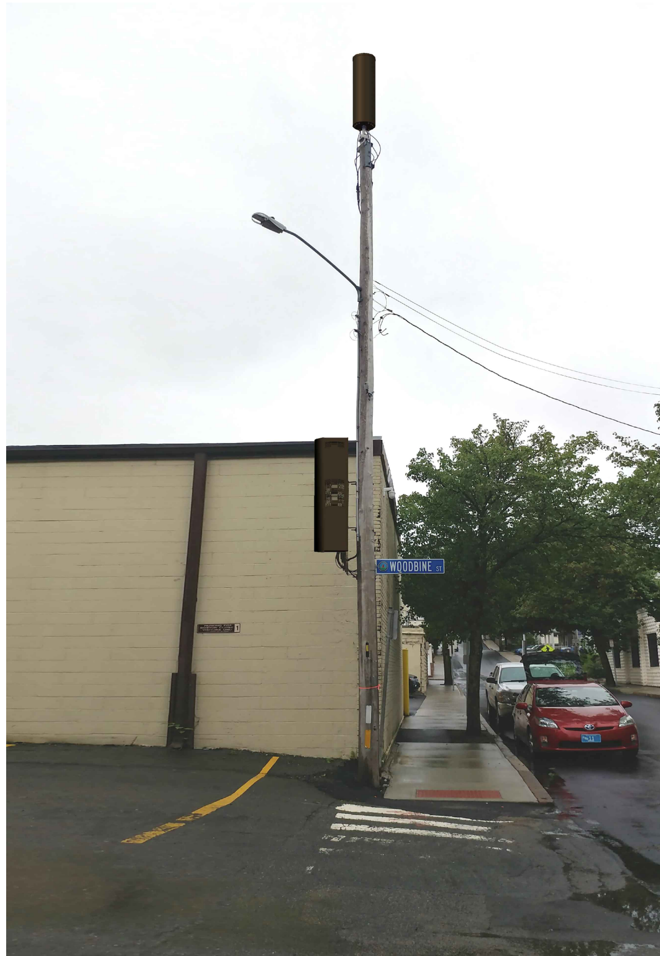
UTILITY POLE – AFTER
