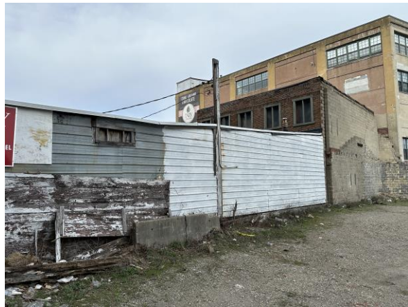
Looking north at subject from adjacent property
