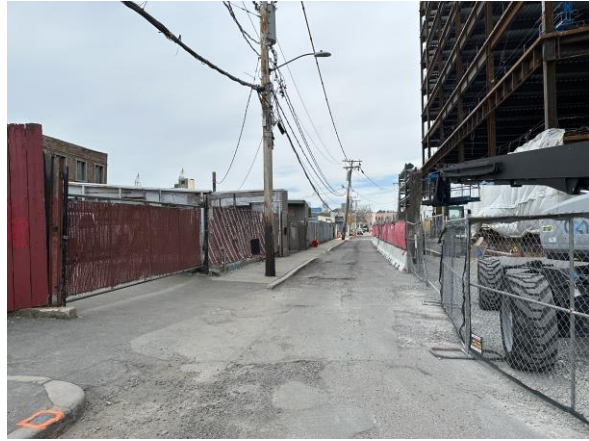
Looking south along Columbia Street, subject on the left
