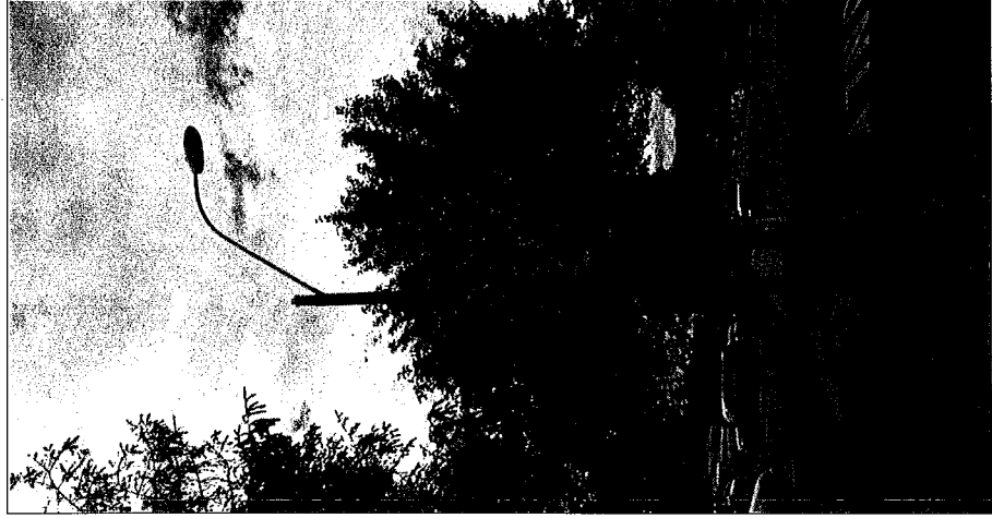
EXISTING LAMP POST LOOKING WEST
