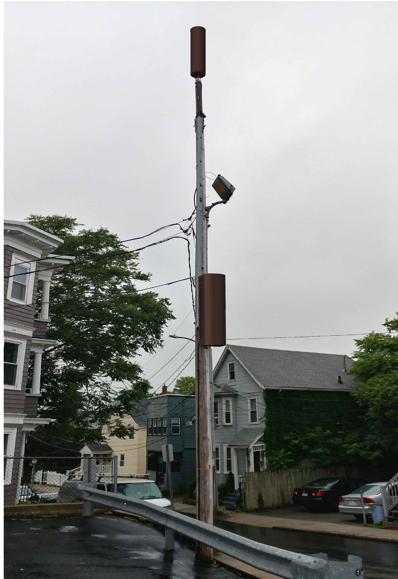
UTILITY POLE – AFTER
